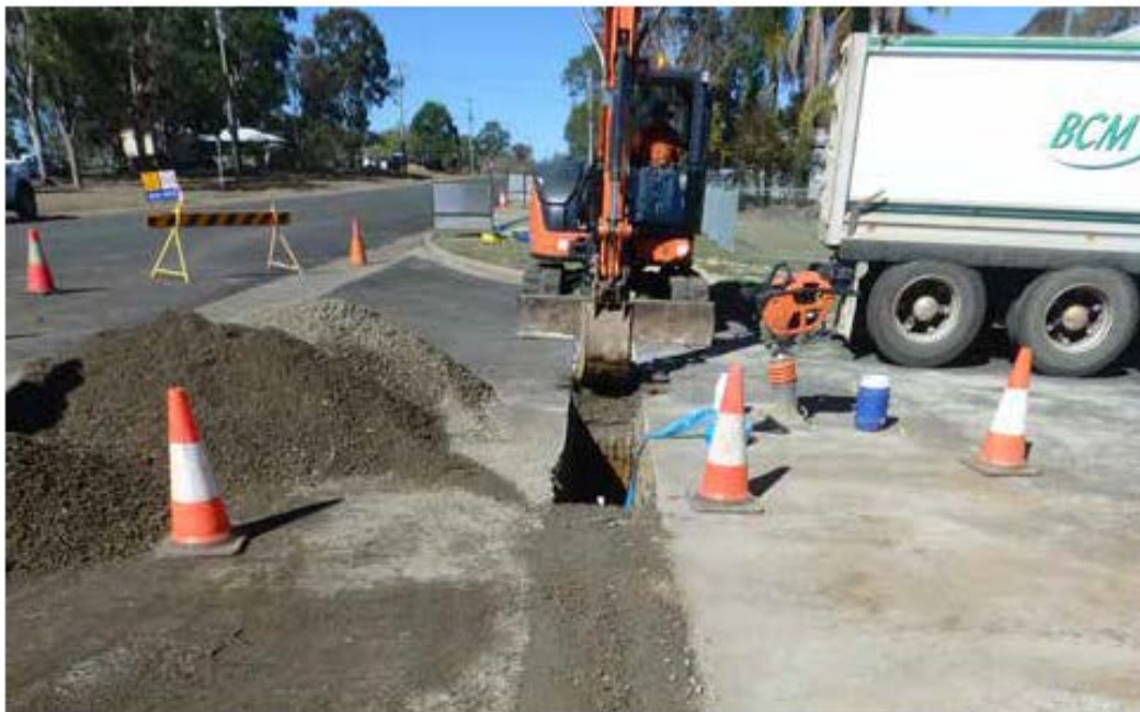
Deakin Crescent, Nanango water main replacement
