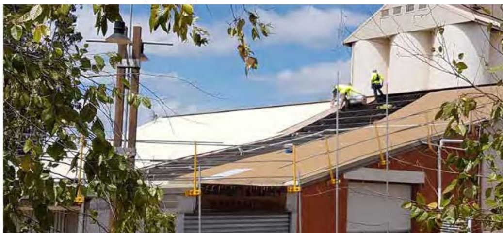
Workers installing the new roof at Kingaroy Heritage Museum
