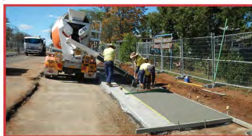
Work undertaken at Durong State School
