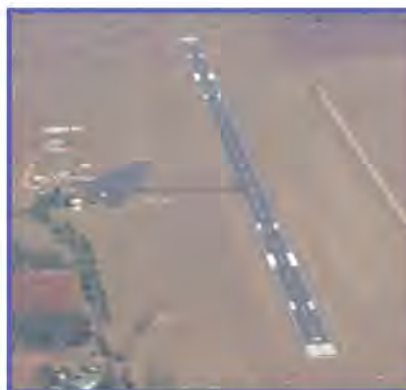
New line marking at the Kingaroy Airport
