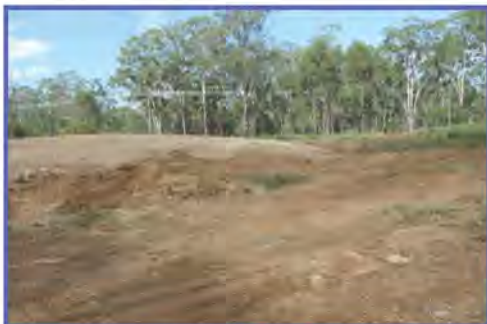
Completed capping of the Wondai Sanitary Disposal Depot
