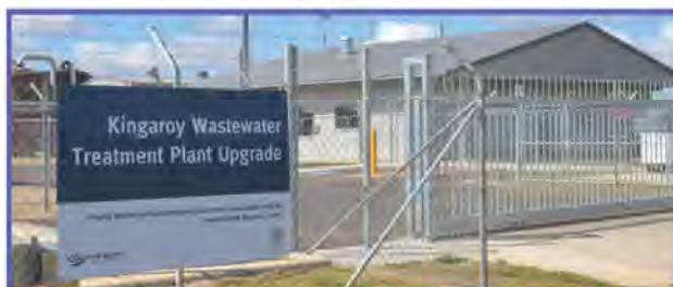
The upgraded Wastewater Treatment Plant [photo courtesy of South Burnett Online]
