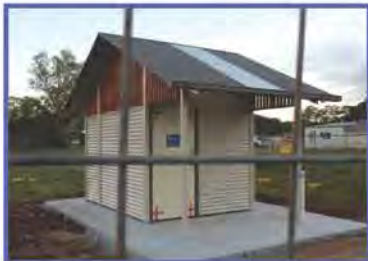
The toilet block at Memerambi nearing completion
