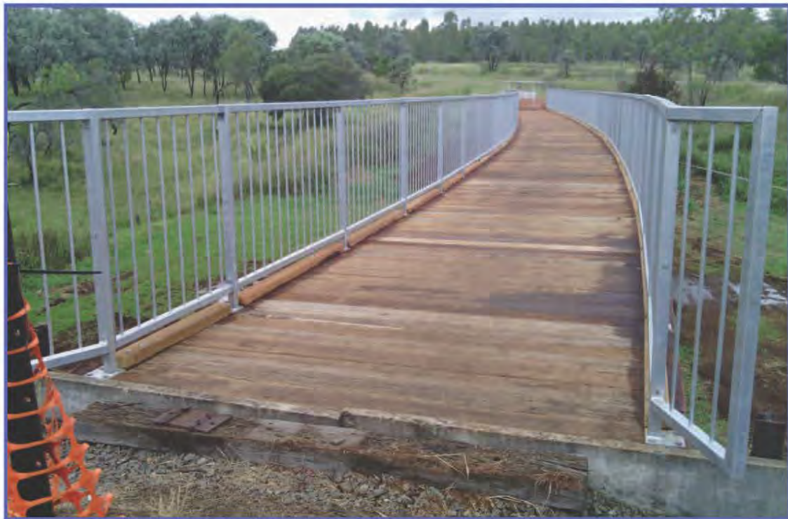
Construction of the Tingoora bridge on the Kilkivan to Kingaroy Rail Trail
