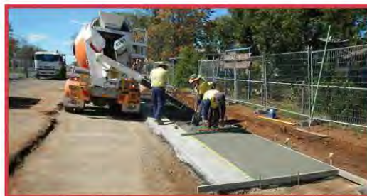
Work undertaken at Durong State School
