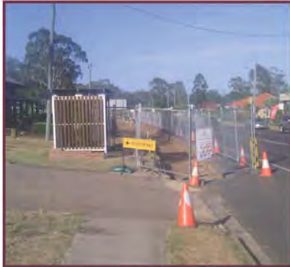
Kerb and channel replacement works at Haly Street, Wondai
