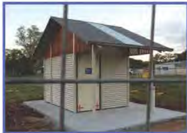
The toilet block at Memerambi nearing completion
