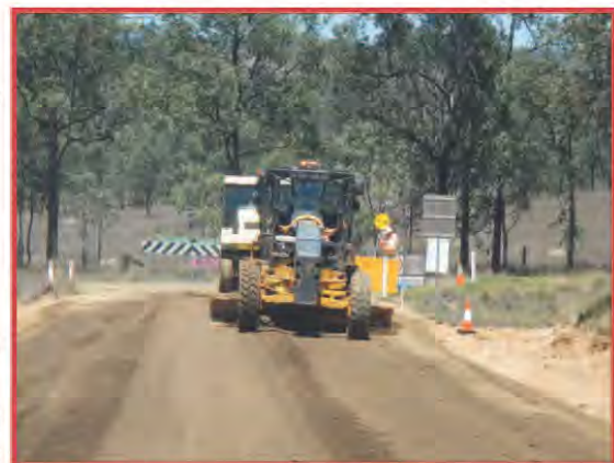
Gravel Resheeting at Hodges Dip Road
