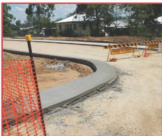
Road construction, kerbing and sealing in Gladys Street, Blackbutt
