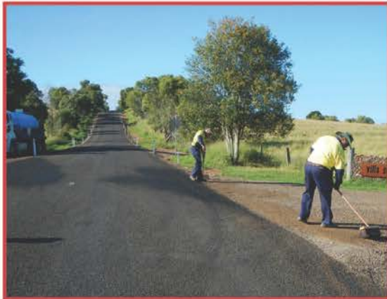
Crest widening at Hazeldean Road, Nanango
