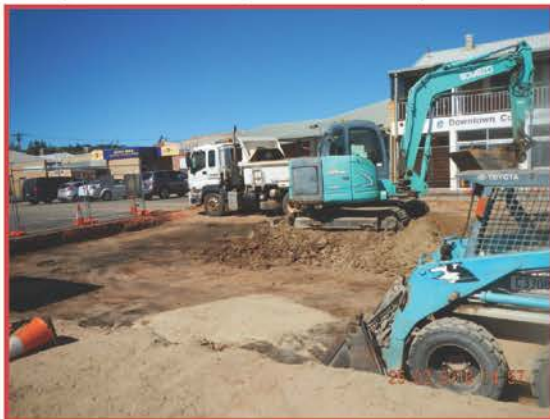
The Glendon Street Car Park upgrade during construction
