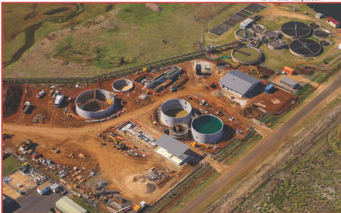
The Kingaroy Wastewater Treatment Plant under construction
