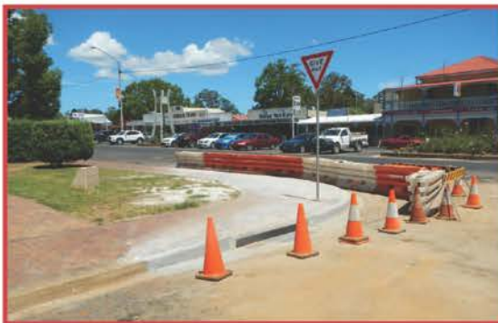
Stormwater upgrade near completion at Coulson Street, Blackbutt
