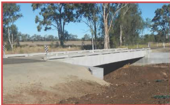
Hansen's Gully Bridge on Mondure Road
