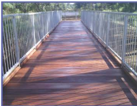
The newly constructed Memerambi North Bridge
