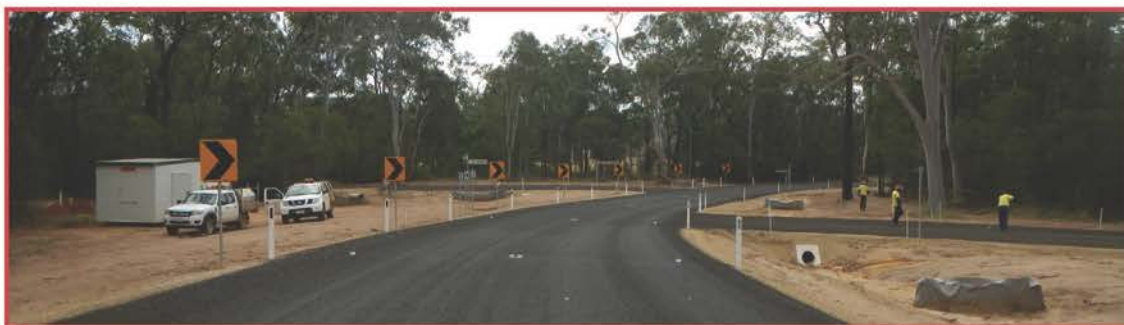
Intersection upgrade at Ellesmere Road, Kingaroy
