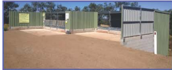
Recently completed Waste Transfer Stations at Durong
