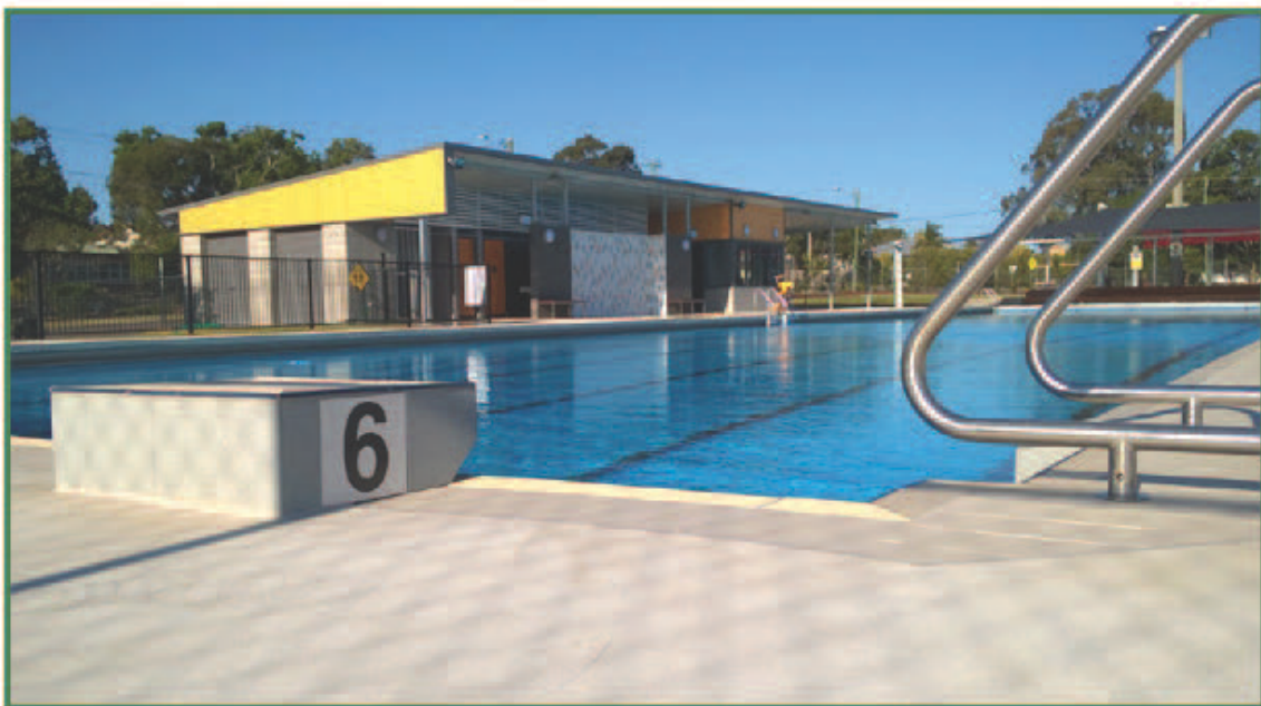
The upgraded Murgon Jubilee Swimming Pool offers a safe and modern environment for patrons
