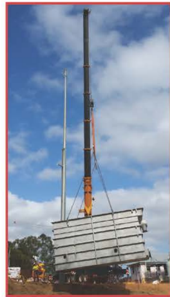
Hams Crane Hire lifting one of three DAFF units into position
