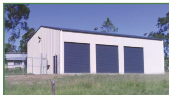
The new SES Storage & Equipment Shed on Grey Street, Nanango
