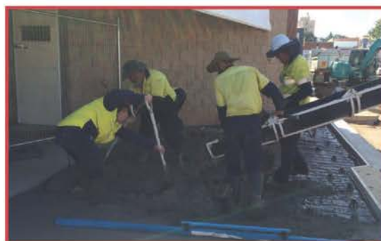
Carpark upgrade at Glendon Street, Kingaroy
