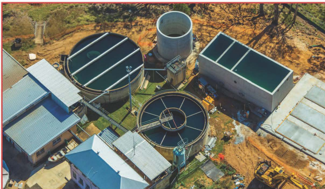
The Gordonbrook Water Treatment Plant under construction
