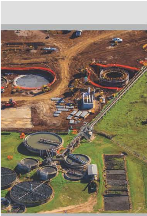
Above: Progress of construction work at the new Kingaroy Wastewater Treatment Plant in April 2014. The existing Kingaroy Wastewater Treatment Plant in the foreground.
