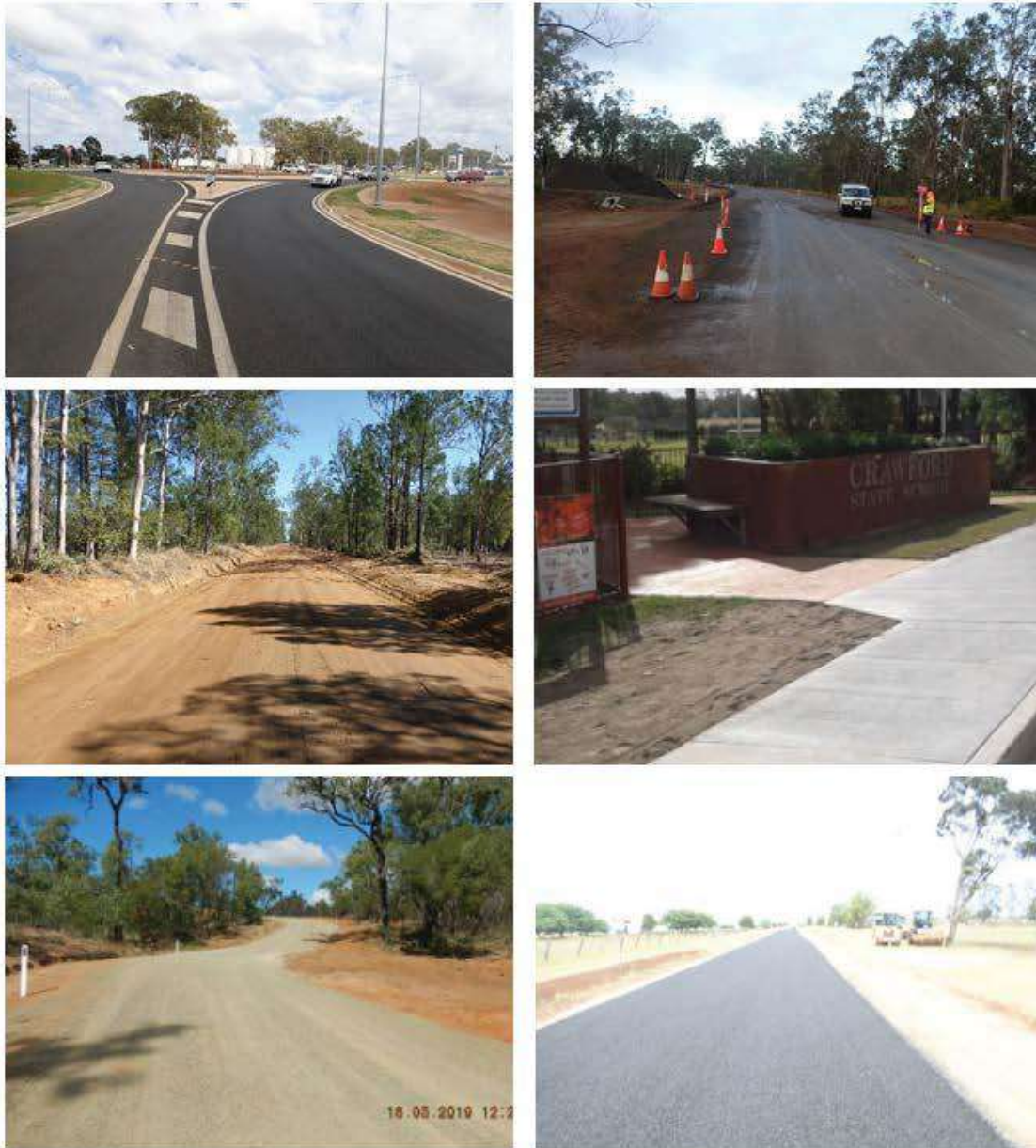
Clockwise from top left: D’Aguilar Highway – Rogers Drive and Industrial Avenue, Construction of a new roundabout (DTMR); Byee Road, Byee, Widen and overlay (DTMR); Siefert Street, Crawford, Crawford State School, Construct Footpath (TIDS); Logan Street, Kingaroy, Reconstruction and Bitumen Seal (RTR); Shellytop Road, Durong, Gravel Resheeting (RTR); Jacksons Road, Durong, Gravel Resheeting (DCP)
