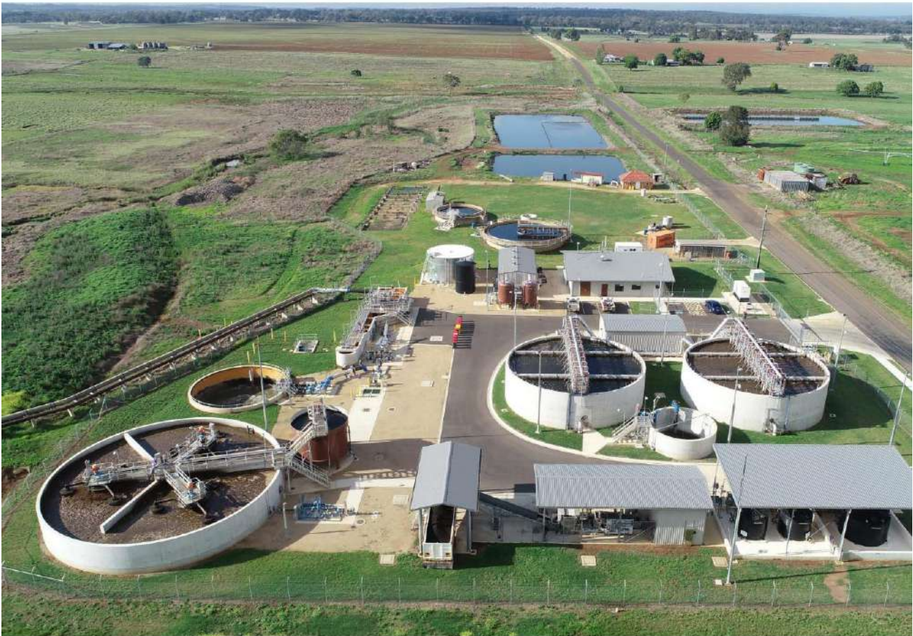
Above: Aerial shot of the Kingaroy Wastewater Treatment Plant
