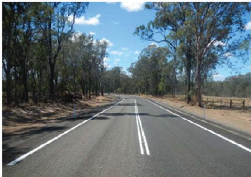
Top: Siefert Street, Crawford, Crawford State School, Construct Footpath (TIDS) Bottom: Memerambi Barkers Creek Road, Memerambi, Road Upgrade (TIDS)
