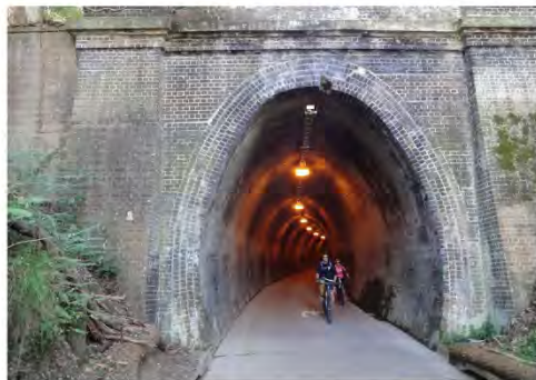
Above: The Fernleigh Track in Newcastle is exceedingly popular with a range of users. One of its key attractions is the Fernleigh Tunnel.
