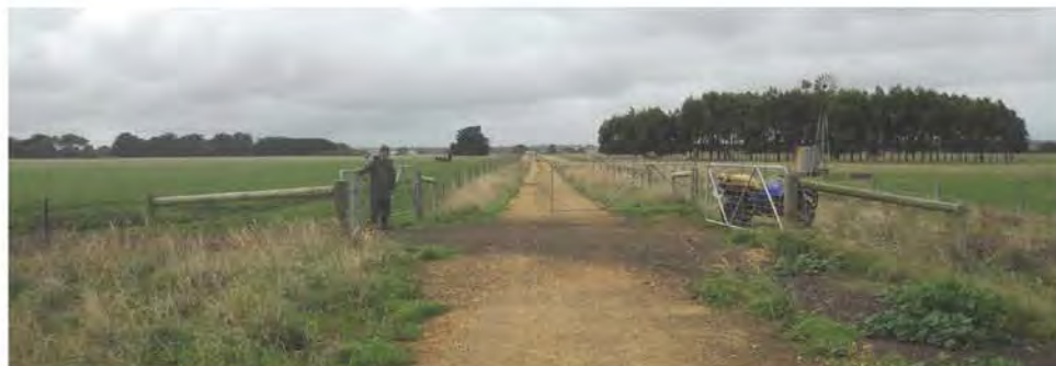
Below: the farmer alongside Port Fairy Warrnambool Rail Trail (in Victoria) has complete control over gates and opens them when he needs to move stock and machinery across the corridor.
