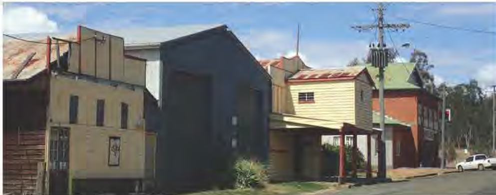
It is possible that development of a trail between Hivesville and Proston may stimulate re-use of these old buildings.
