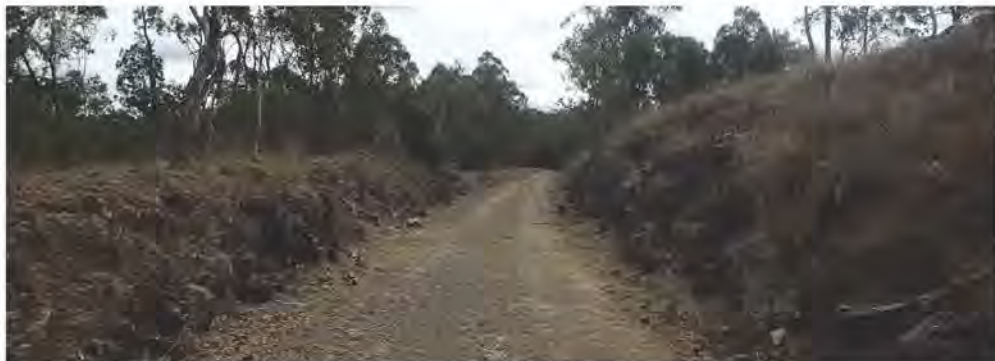
Arrangements would need to be made to keep motor vehicles off the formation should a trail be constructed.
