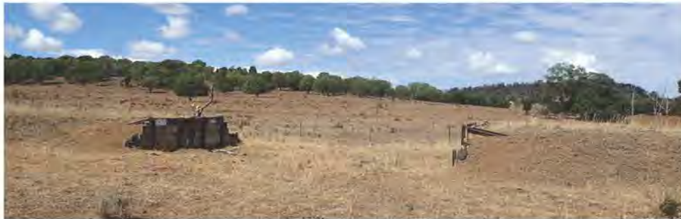
Apart from the abutments, very little remains of the original bridges along the former railway corridor.
