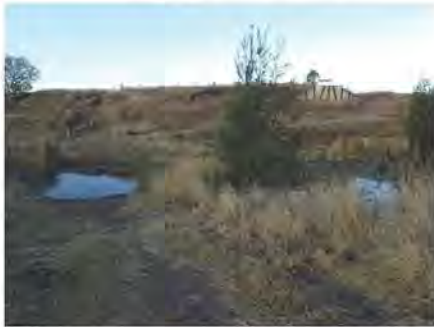
Above: A flooded waterway crossing on the Kingaroy Kilkivan Rail Trail.
