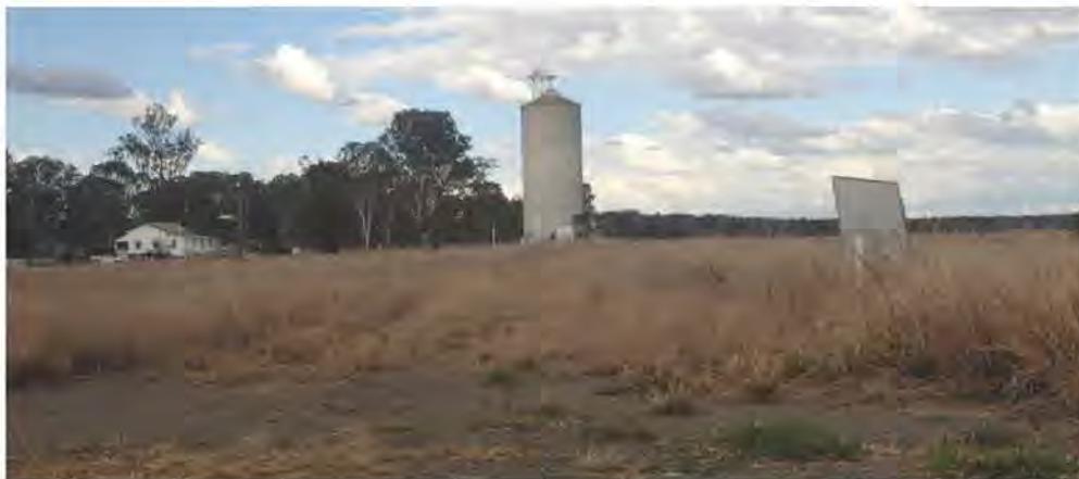
As with many of the small sidings on this corridor, no physical evidence of Byee siding remains.
