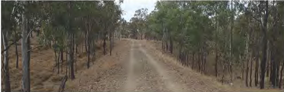
Cuttings and embankments are present on this section and one of the features rail trail users look for. It can be seen that the corridor is already in use for vehicle access. With good design, this access can be retained.
