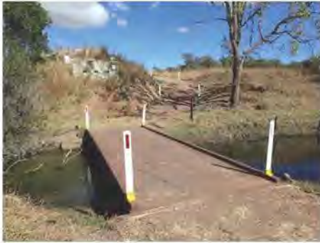
Above: A low level timber bridge across a creek on the Kingaroy Kilkivan Rail Trail.
