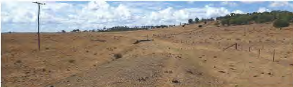
Much of the corridor is unfenced and vegetation has been removed.
