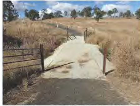
Above: A concrete floodway across a creek on the Kingaroy Kilkivan Rail Trail.
