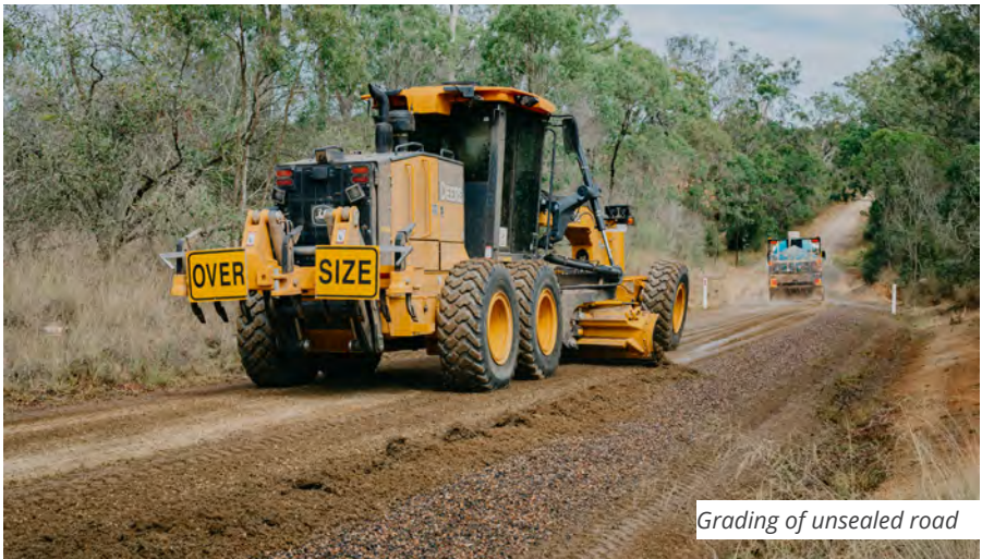
Bunya Avenue - Bunya Mountains Bitumen Reseal
