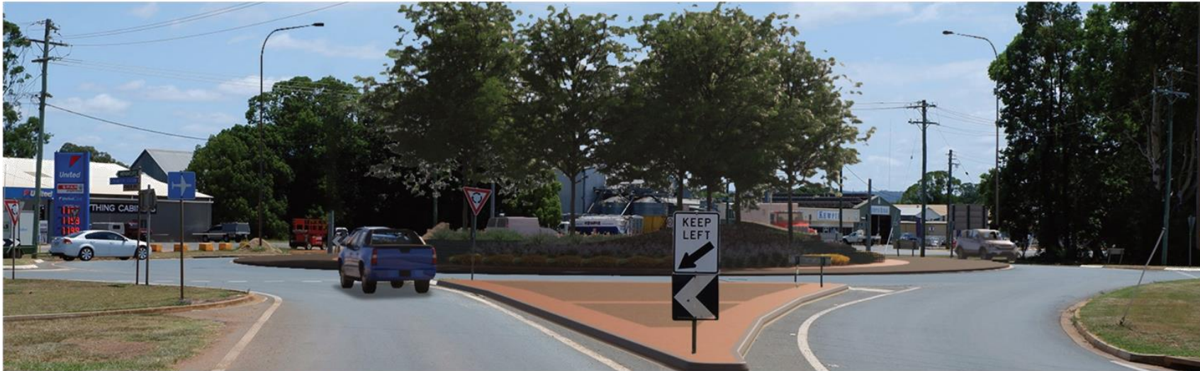
YOUNGMAN STREET & RIVER ROAD ROUNDABOUT LOOKING NORTH
