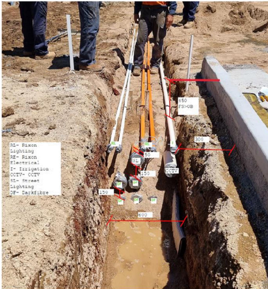
Image of Alford St Conduit Bundle – at Shopping Work Entrance
