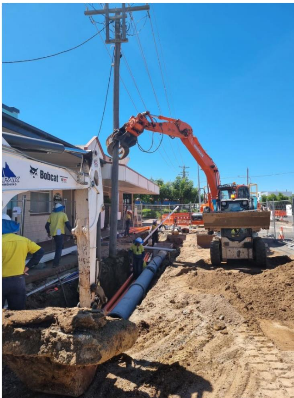
Image of Ergon approved Safety works – whilst laying conduits and stormwater
