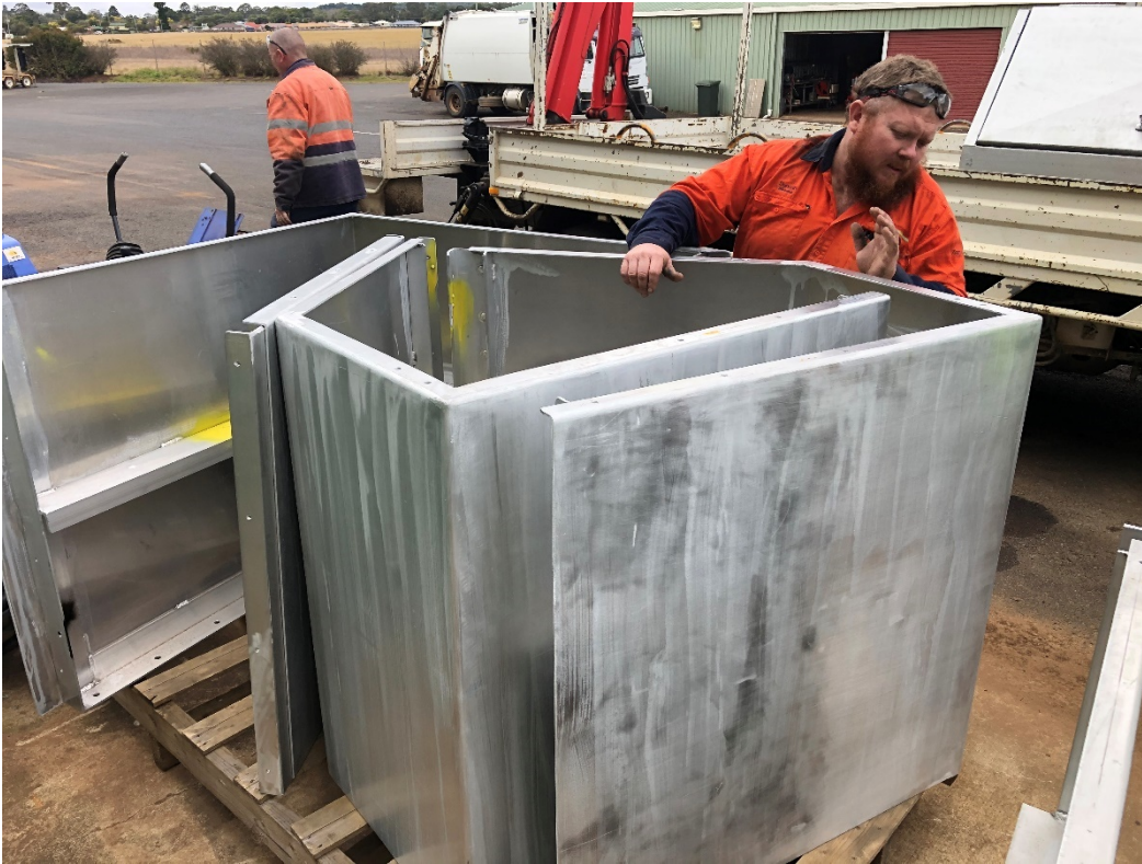
Image of part of the internal concrete mold for the raised planters fabricated by SBRC workshop team for use in next stage works
