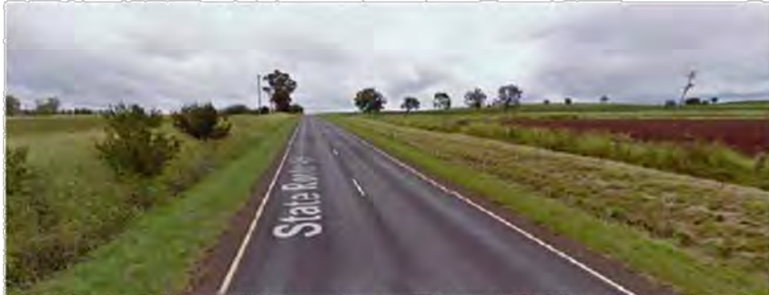
Figure 2-3: Bunya Highway typical cross section, East of Mannuem Road facing West (Google Maps Street View)
