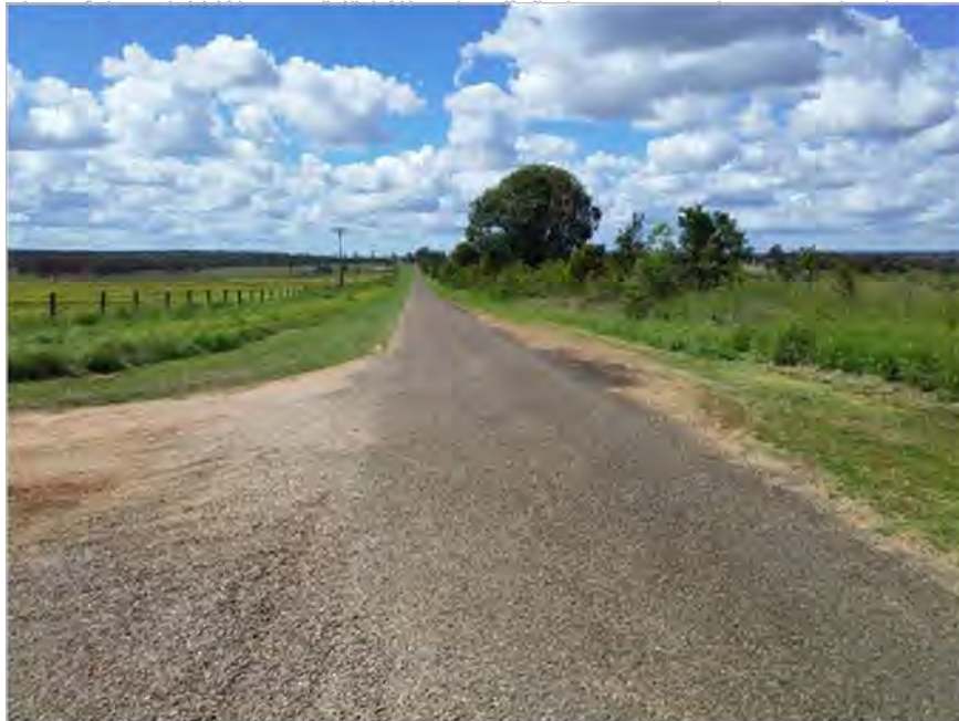
Figure 5-5: Sight distance on Mannuem Road looking North
