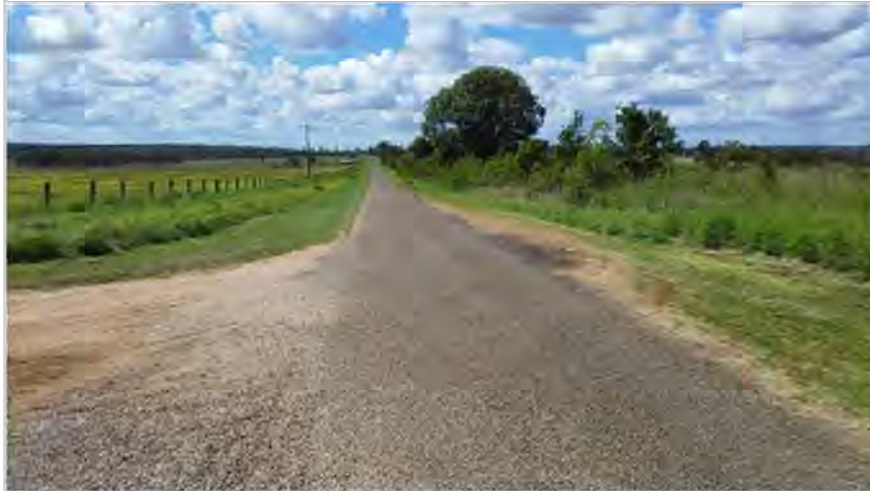
Figure 2-2: Mannuem Road typical cross section, looking North from the development site access
