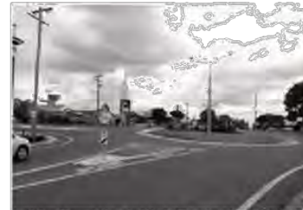
Existing Roundabout at Malby Street and Scott Street, Wondaí
