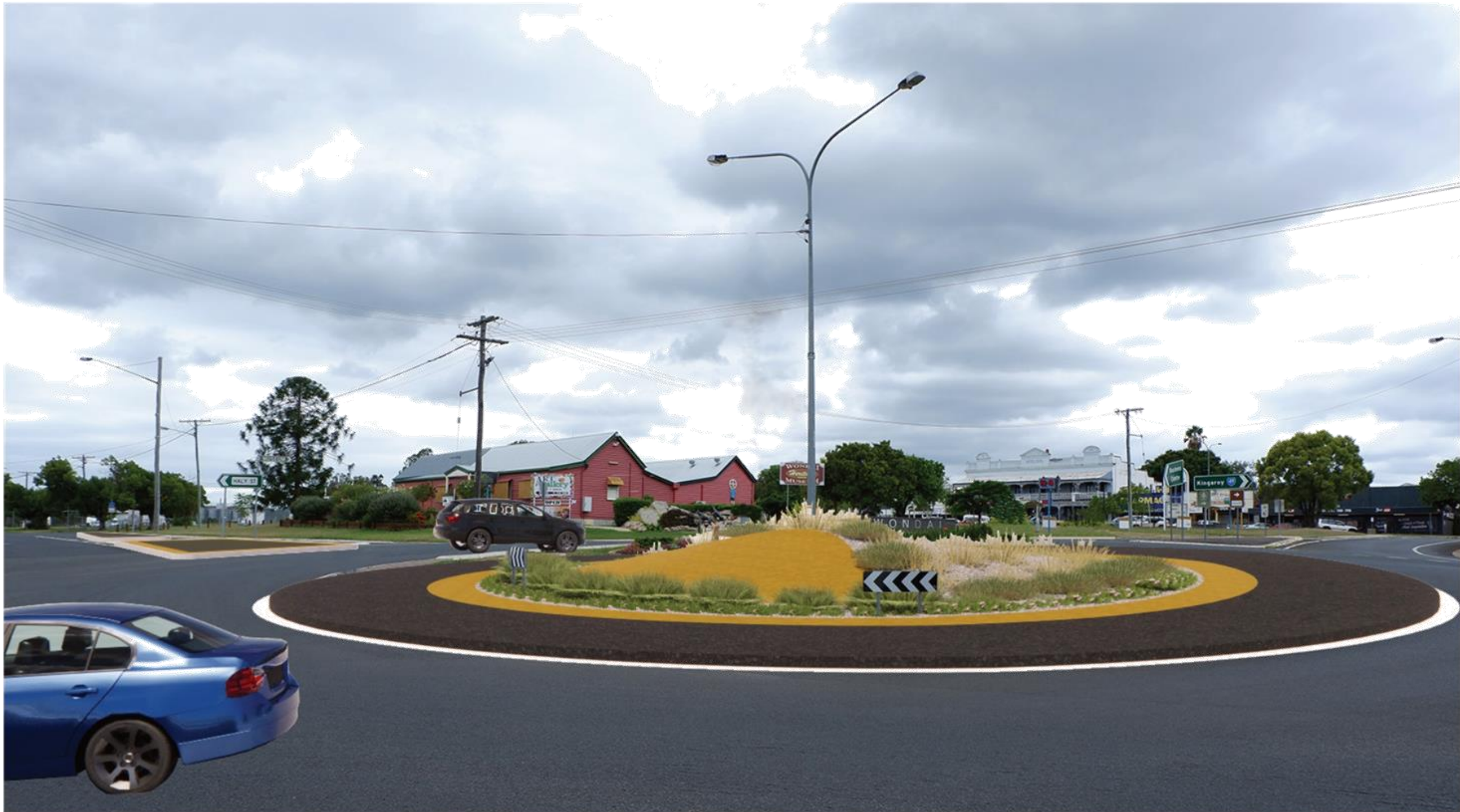
HALCYON STREET & SCOTT STREET ROUNDABOUT LOOKING SOUTH TOWARDS THE ART GALLERY
