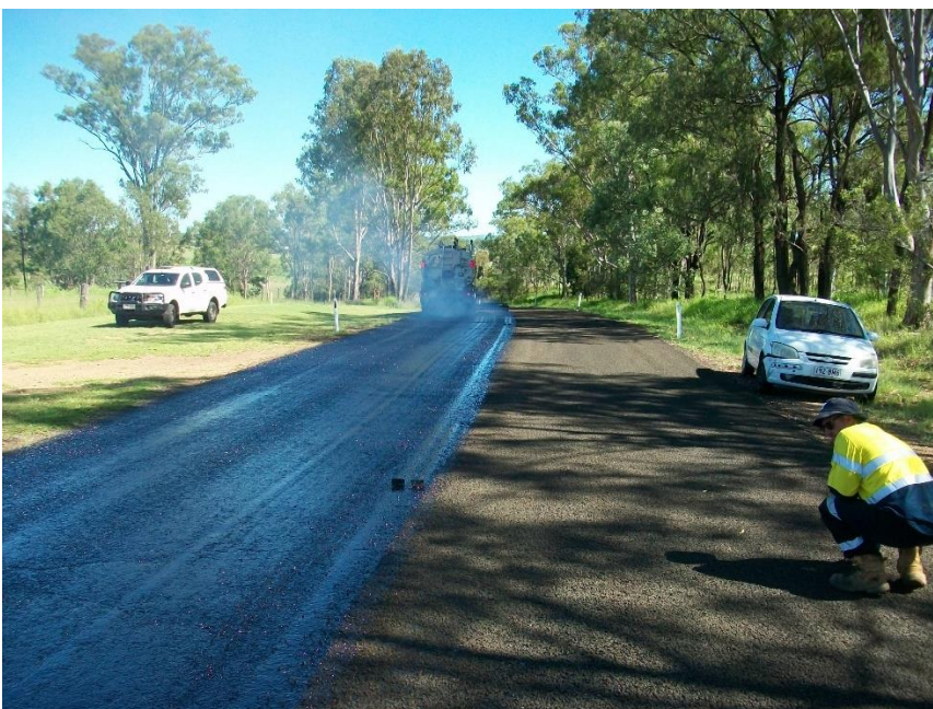
Bitumen Resealing Cherbourg Road following various maintenance repairs.
