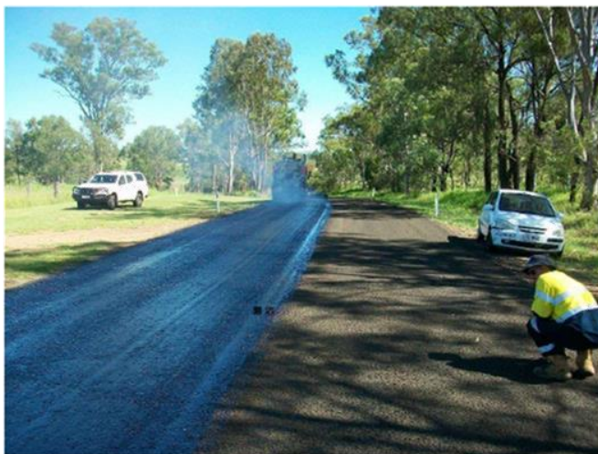
Bitumen Resealing Cherbourg Road following various maintenance repairs.
