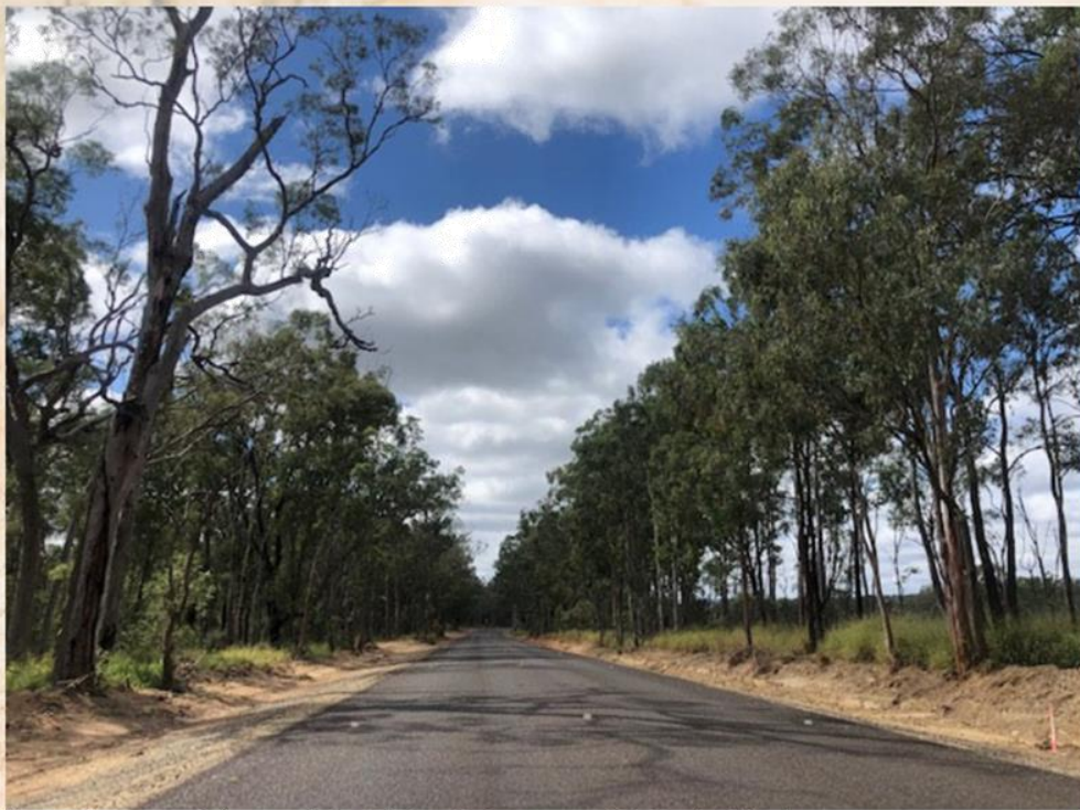
Figure 1- Recent upgrade from unsealed to sealed standard on Memerambi Barkers Creek Road
