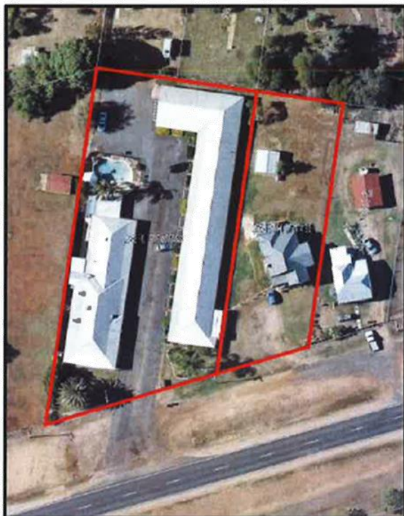
Figure 1 - Aerial Image (Source: Qld SPP mapping)
