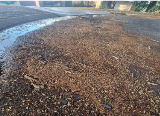
Tree droppings clogging the stormwater pit following rain event at Leopard Court
