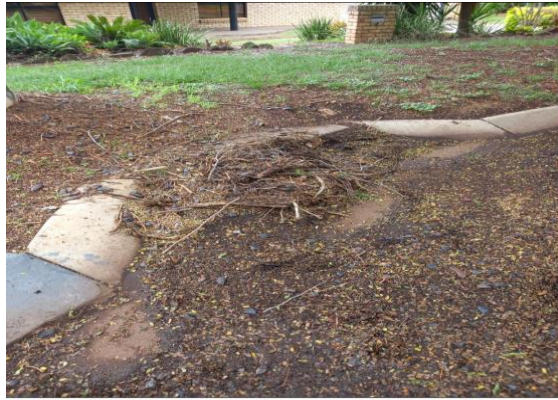
Tree droppings clogging the stormwater pit following rain event at Leopard Court
