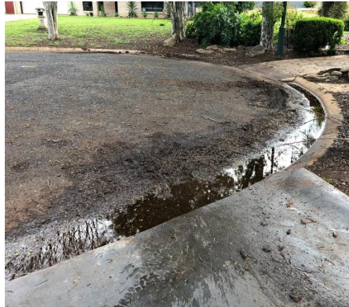
Tree droppings clogging the stormwater pit following rain event at Leopard Court
