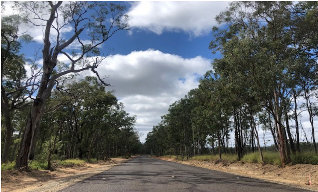
Figure 1- Recent upgrade from unsealed to sealed standard on Memerambi Barkers Creek Road
