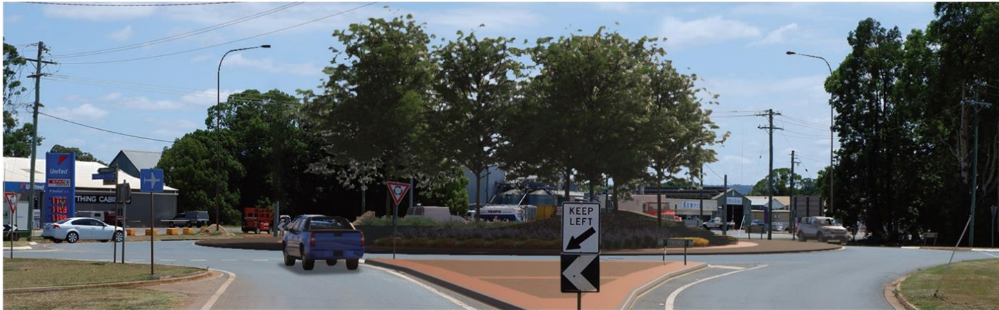
YOUNGMAN STREET & RIVER ROAD ROUNDABOUT LOOKING NORTH
