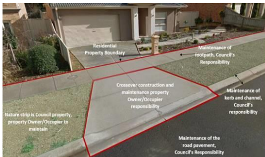
An example of a residential property access and kerb crossover
