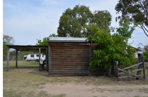
Figure 176. The north-west elevation of the postal receiving office, showing the thin chamferboards used in the c.1950s construction of the carport extension.
