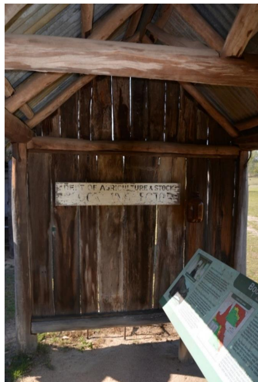
Figure 208. Interior of the DPI shelter, showing the existing interpretation signage.
