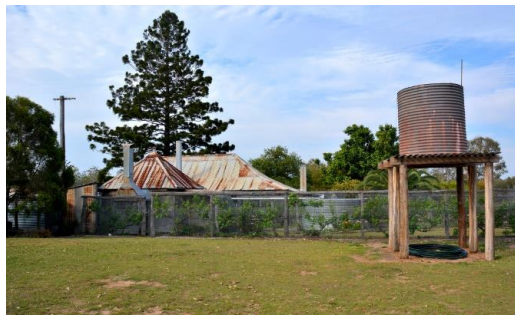
Figure 60. View facing east of the rear elevation of the main homestead from the open space between the cluster of other historical structures.
