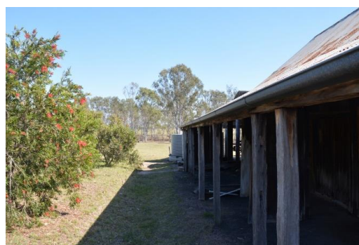
Figure 138. View facing north-west along one of the lean-to verandah additions to the stone store.
