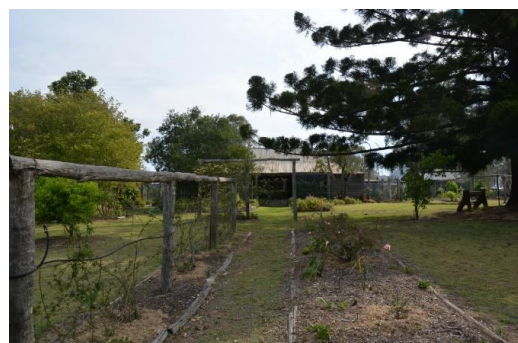
Figure 57. Long view of the entrance to and principal elevation of the main homestead eastern entrance from within the homestead’s gardens.
