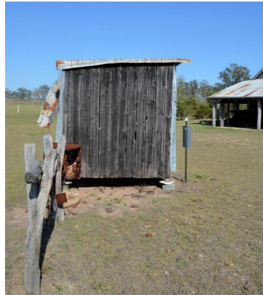
Figure 210. The eastern elevation of the boundary rider's hut, with the stone store building partially visible at the right.
