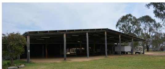
Figure 228. The north-eastern elevation of the ‘Big Top’ extension.
