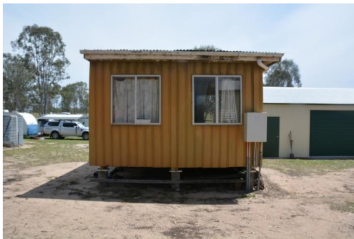
Figure 217. The north-eastern elevation of the archives building.
