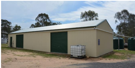
Figure 266. The south-east elevation of the shed.
