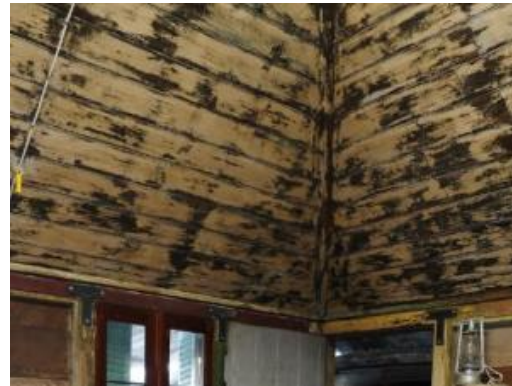
Figure 127. Detail of the ceiling of the detached kitchen, lined on the rake with unpainted, horizontally-fixed beaded boards.
