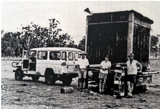
Figure 30. Lionel, Helen, and Phill pose in front of the structure known as the boundary rider's hut following its relocation to Boondooma, where it was re-stumped. Source: Boondooma Museum & Heritage Association (2021) 54
