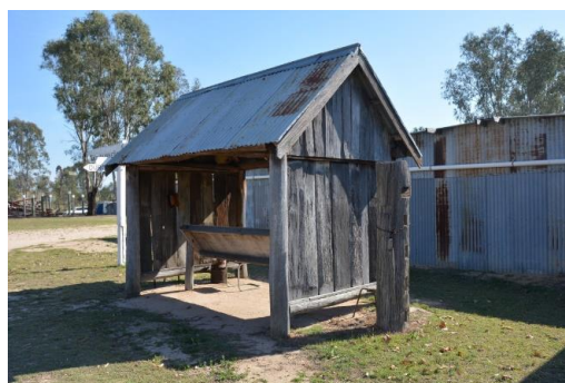
Figure 206. The south-west elevation of the DPI shelter, showing the remnant timber post of the cattle dip installed herein 2006 known as 'Stockie's Stump'.
