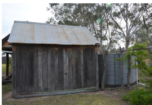
Figure 151. The north-east elevation of the meat house with a large water tank adjacent.
