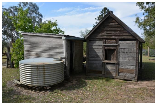
Figure 171. The rear south-west elevation of the postal receiving office, showing the adjacent airport skillion-roof extension and water tank.
