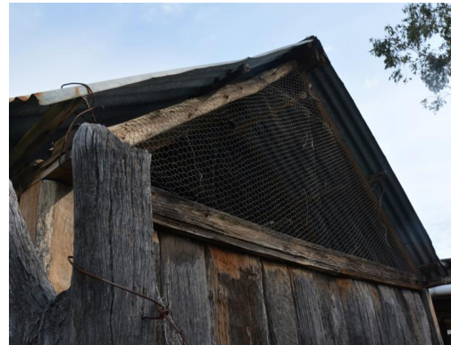
Figure 156. Detail of the chicken wire mesh gable infill.
