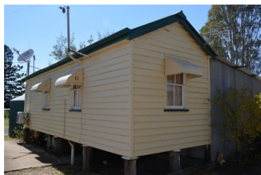
Figure 216. The south-western corner of the administration building.
