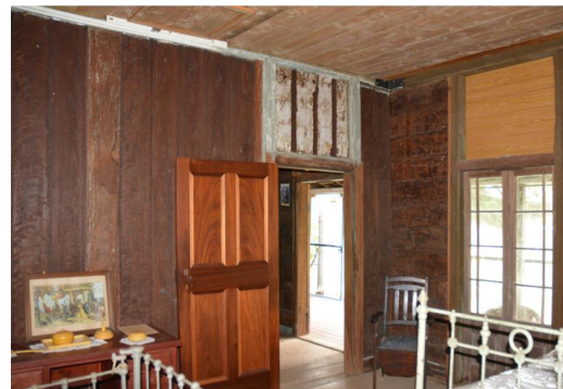
Figure 109. Interior of Bedroom 1.
