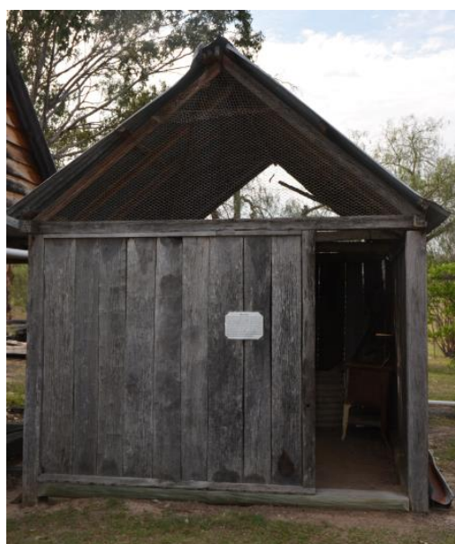
Figure 152. The main south-east elevation of the meat house.
