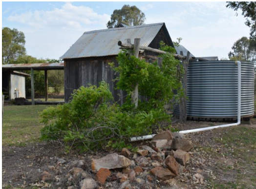
Figure 155. View facing south-west of the meat house, showing the adjacent water tank and timber trestle supporting the rainwater goods.
