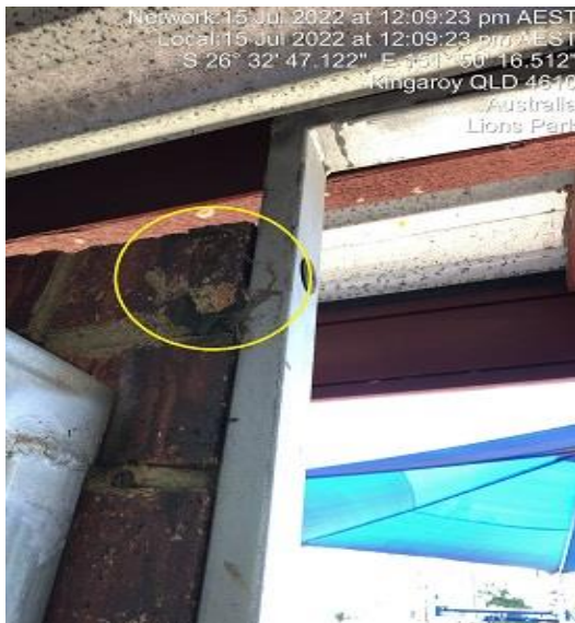
Damaged brickwork
