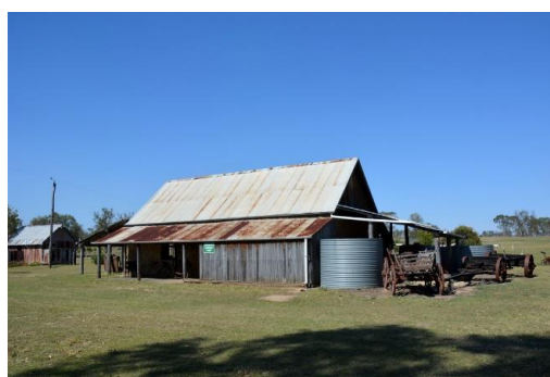
Figure 134. View facing south-west of the stone store building.
