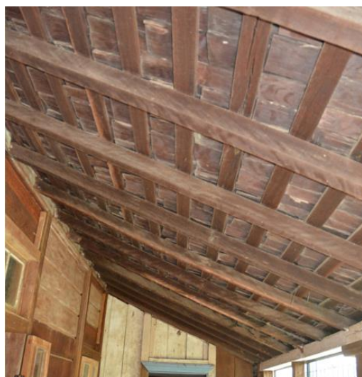
Figure 90. The underside of a section of the front verandah roof, showing the early timber shingles.
