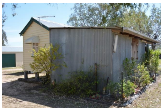
Figure 215. The south-eastern corner of the administration building, showing the corrugated iron skillion extension.
