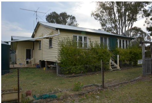
Figure 189. The south-east elevation of the caretaker's cottage.
