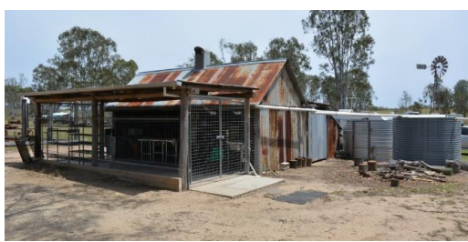
Figure 247. The south-eastern elevation of the camp kitchen.
