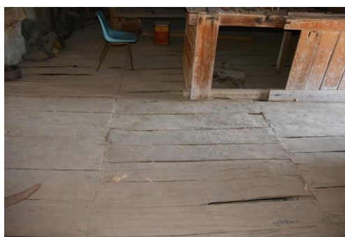
Figure 146. Interior view of hardwood shot-edge boards of the Stone Store.
