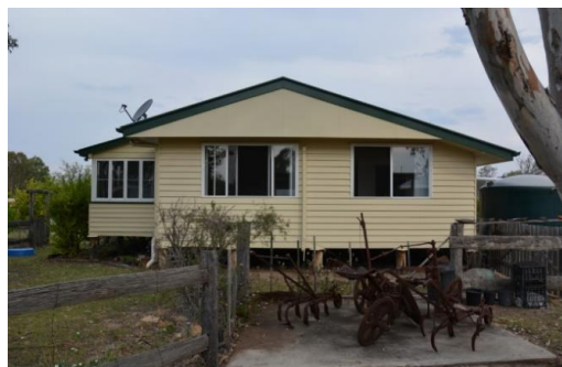
Figure 192. The south-west elevation of the caretaker's cottage.
