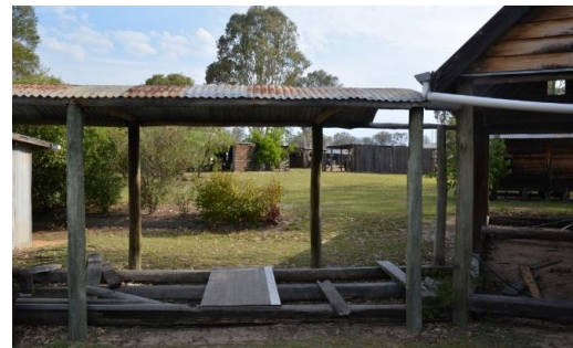
Figure 61. View towards the cluster of other historical structures from the covered walkway of the main homestead.
