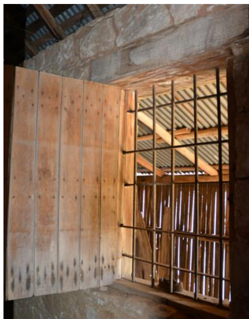
Figure 150. Detail of a typical window shutter made of vertical timber slabs.
