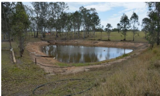
Figure 268. View facing north-west of the dam located on the Boondooma Homestead property.
