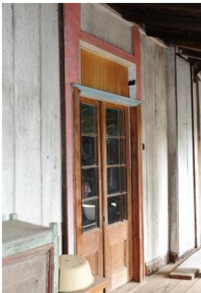
Figure 96. Example of the timber French doors leading from the main bedroom onto the rear verandah, noting the infilled fanlight.
