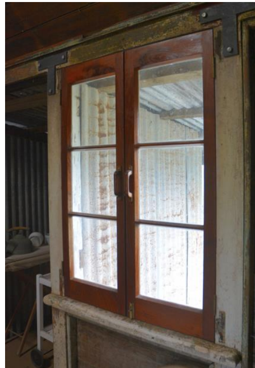
Figure 125. Example of the replacement timber casement windows in the kitchen, which are non-sympathetic additions.
