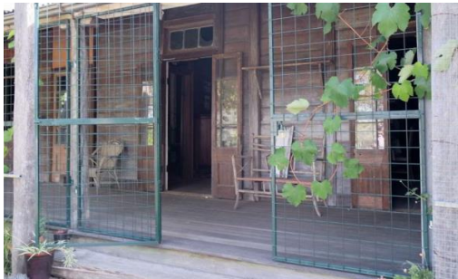
Figure 88. The front verandah of the main homestead, showing the modern, powder-coat steel, grid-mesh screening that encloses the verandah for security purposes.
