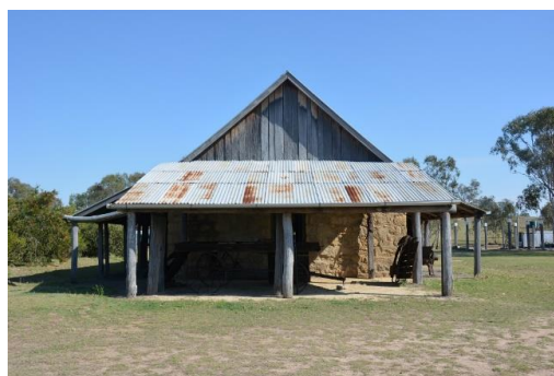
Figure 132. The south-east elevation of the stone store building, where the lean-to verandah addition is utilised for the display of a historical wagon.
