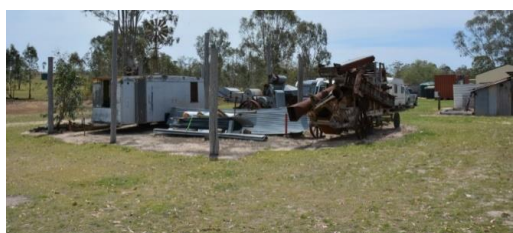
Figure 252. The south-western corner of former machinery shed.
