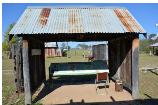
Figure 205. The north-east elevation of the DPI shelter.
