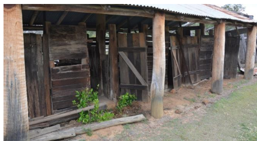
Figure 186. The timber slabs doors that divide the milking bails structure internally to create individual stalls.
