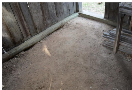
Figure 154. Interior of the meat house showing the compacted earth floor.
