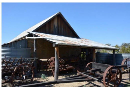
Figure 137. The verandah on the north-west elevation of the stone store building, used to display associated machinery pieces.
