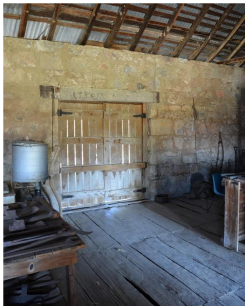
Figure 148. Interior view of the south-west wall of the stone store, showing the floor constructed of wide, hardwood shot-edge boards atop timber joists and bearers, which were restored and reconstructed in the early 2000s.
