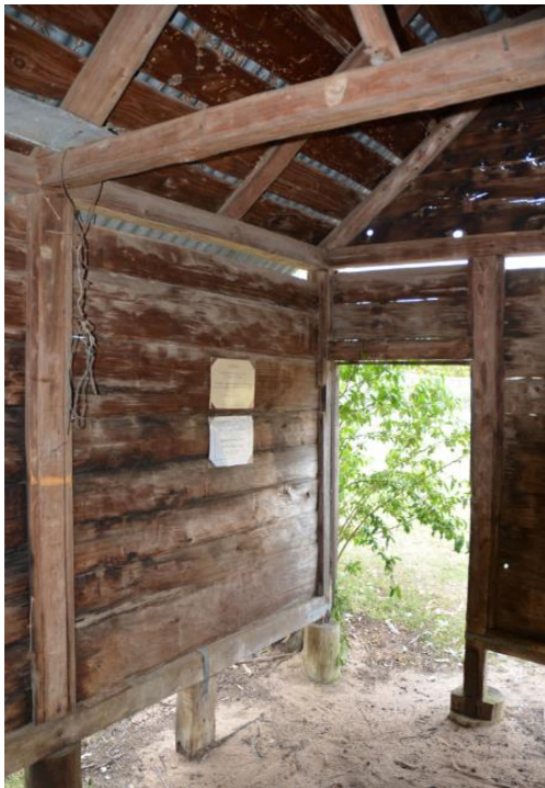
Figure 167. Interior of the cool house, illustrating its construction of horizontal timber slabs of Cypress pine.
