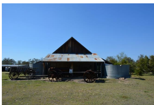
Figure 133. View of the north-west elevation of the stone store building, noting the two water tanks attached either side of the structure.
