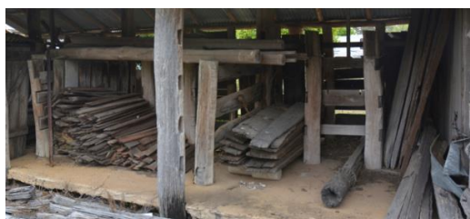
Figure 187. Typical interior view of the milking bails structure, which is not readily accessible due to the use of the structure for storage of timber.
