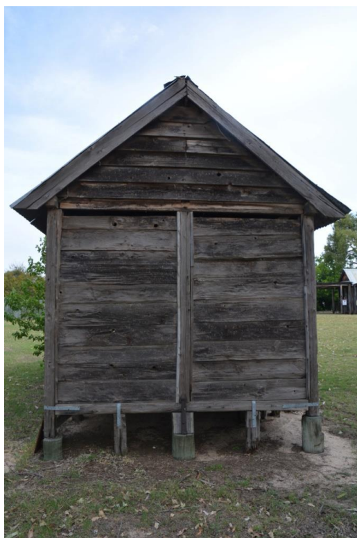
Figure 163. The rear north-west elevation of the cool house, which has been re-stumped in recent years.
