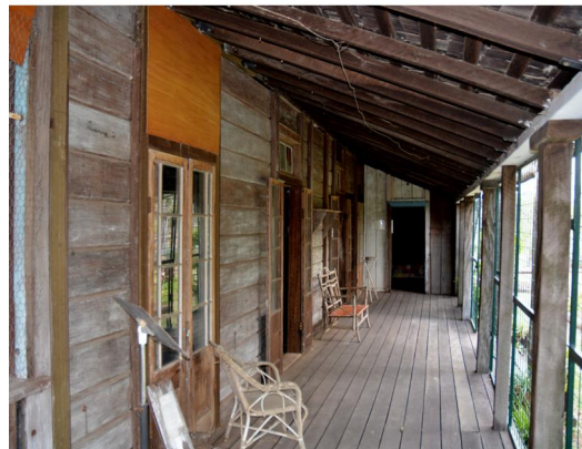
Figure 89. View along the front verandah of the main homestead, showing the French timber doors providing access to the core internal rooms (left) and the bedroom created by the enclosure of the verandah at its western end.
