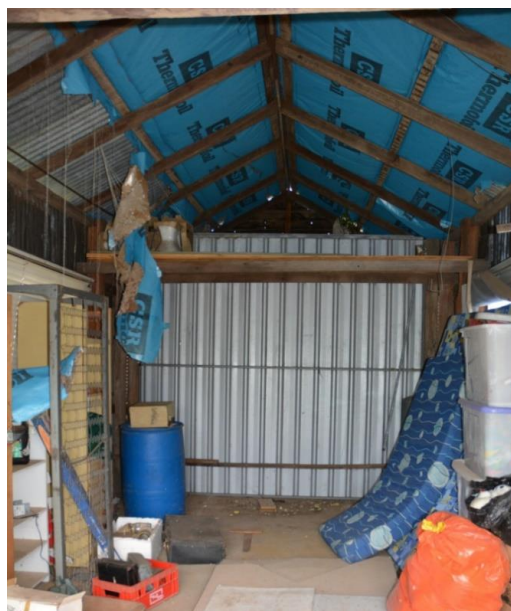
Figure 198. Typical interior of the caretaker's store.
