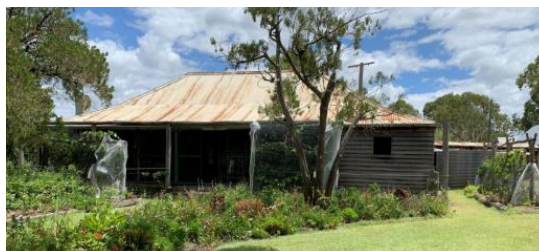
Figure 81. The north-east (front) elevation of the main homestead.
