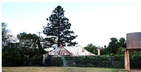
Figure 80. The south-west (rear) elevation of the main homestead.
