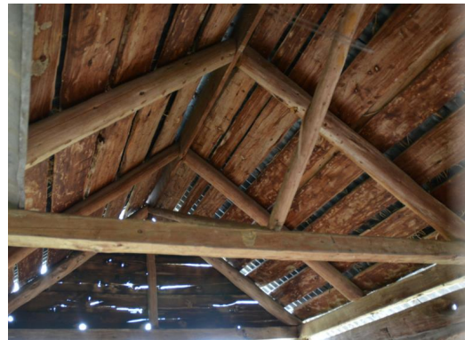
Figure 168. Interior of the cool house showing the gable roof form and horizontal timber slabs of Cypress pine.
