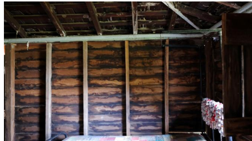
Figure 119. Interior of Bedroom 3 showing the single-skin construction framing exposed in this room.
