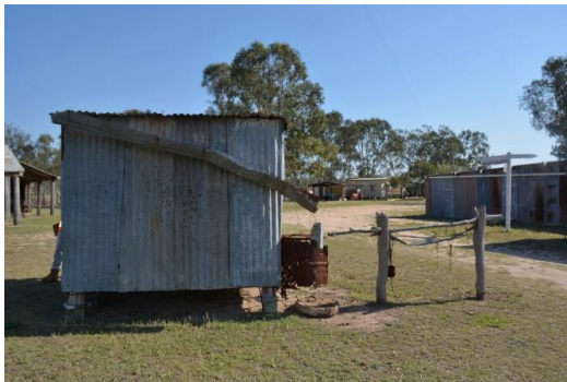
Figure 211. The southern elevation of the boundary rider's hut.
