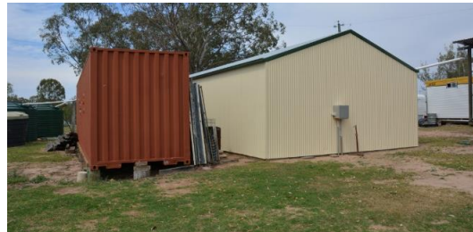
Figure 267. The south-west elevation of the shed, showing the shipping contained installed adjacent at the rear.
