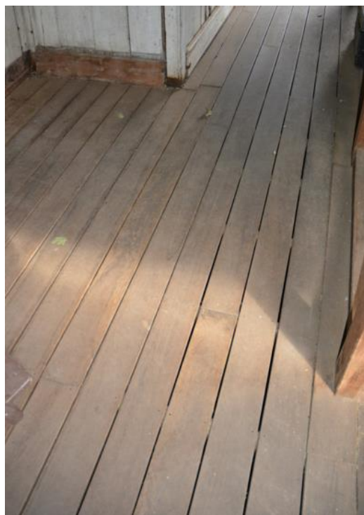
Figure 101. Example of the typical verandah floorboards on the homestead's verandahs, which is lined with shot-edge boards.
