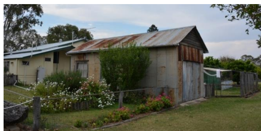
Figure 196. View facing north of the caretaker's store, with the caretaker's cottage visible adjacent in the left background.
