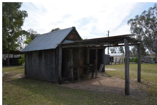
Figure 172. The south-east elevation of the postal receiving office, showing the c.1950s skillion awning attached to the front.
