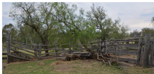
Figure 184. The dilapidated cattle-loading dock, which has a few pepperina plantings either side.
