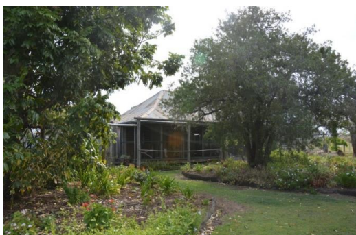
Figure 56. View facing north-west towards the principal elevation of the main homestead from within the homestead’s gardens.
