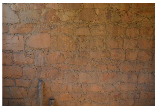
Figure 140. Detail of the typical stonework held together with ant bed mortar.
