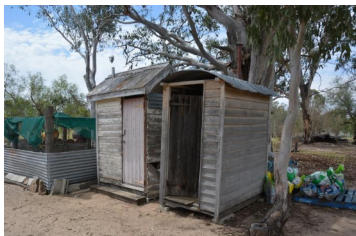
Figure 258. The two timber outhouses.
