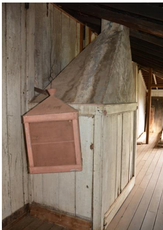
Figure 100. Detail of the exterior of the dining room fireplace, which projects into the verandah space on the south-west of the homestead.
