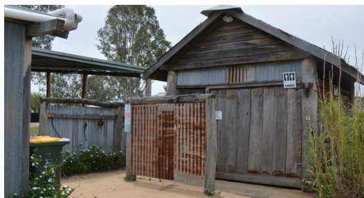
Figure 263. The south-west elevation of the toilet block located adjacent to the 'Big Top' extension.
