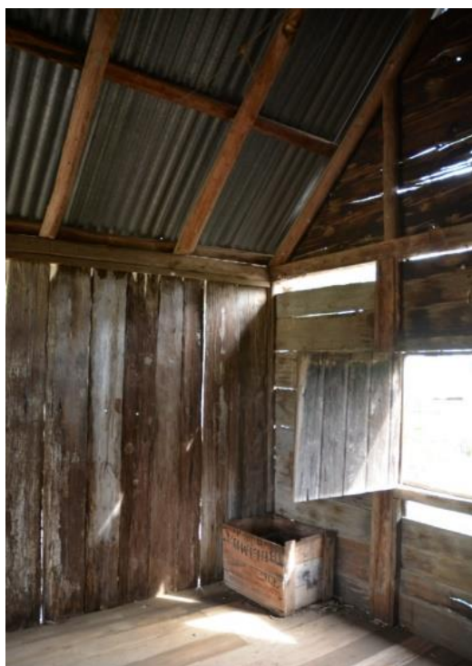
Figure 173. Interior of the postal receiving office, showing the timber slab case window in the rear elevation.
