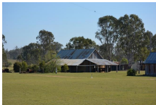
Figure 130. View facing north-west of the stone store building, with one of the toilet blocks partially visible at the right.
