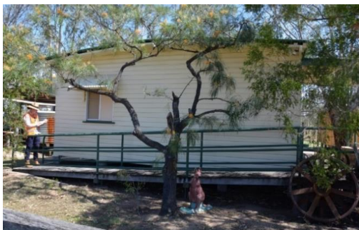
Figure 226. The south-eastern elevation of the museum building, showing timber-framed ramp providing disabled access.
