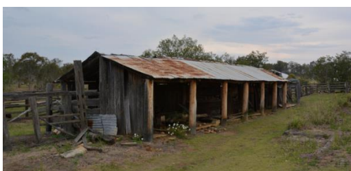
Figure 181. The north-west elevation of the milk bails structure.
