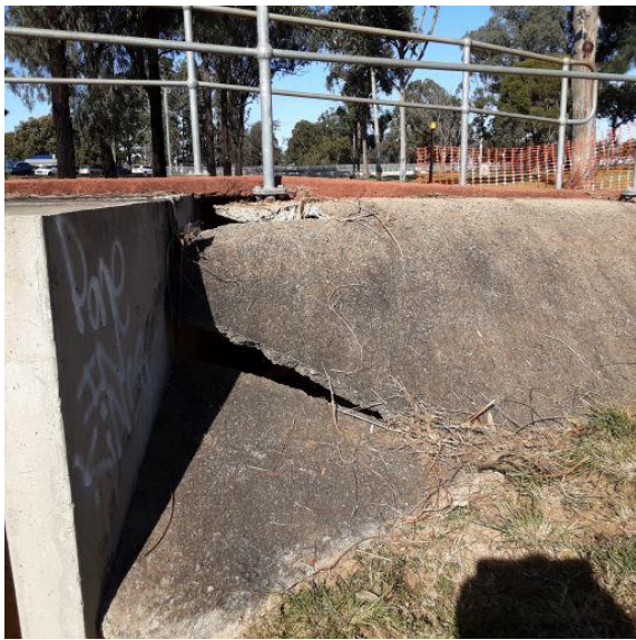
Accessed damaged to bridge damaged from weather event
