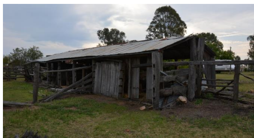
Figure 185. View facing west of the milking bails structure from within the stockyards.
