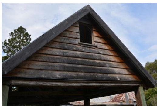
Figure 161. Detail of the timber gable infill.
