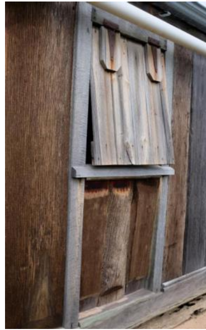
Figure 95. Example of the reconstructed timber window awnings fitted to window openings on the homestead's north-west elevation.
