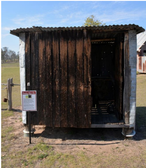
Figure 209. The northern elevation of the boundary rider's hut.
