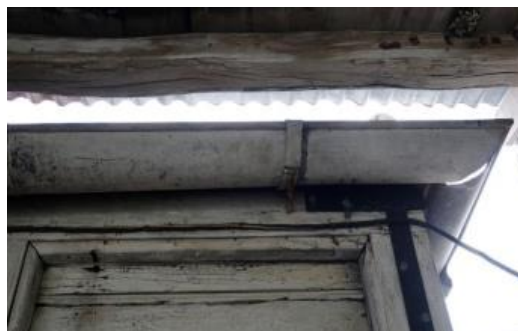
Figure 99. Detail of the half round gutters surviving attached to the northern wall of the homestead's detached kitchen.
