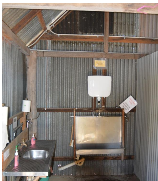
Figure 265. Interior of a typical hand washing area in the toilet blocks.
