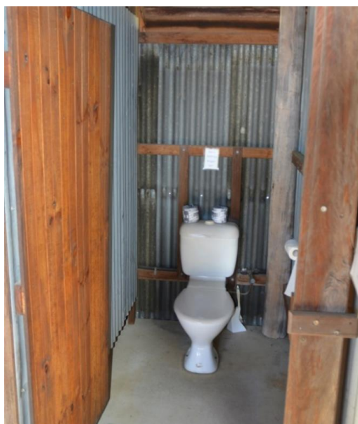
Figure 264. Interior of a typical toilet stall in the toilet blocks.
