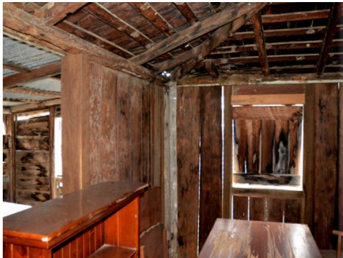
Figure 122. Interior of a small room referred to as a study, adjacent to Bedroom 3.
