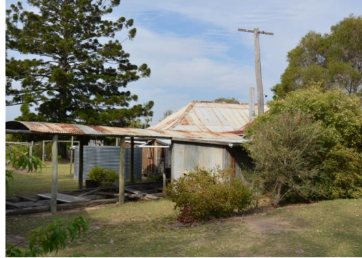
Figure 87. View facing north-east showing covered walkway, constructed of a post-and-sapling frame with a corrugated iron roof, connected to the main homestead.
