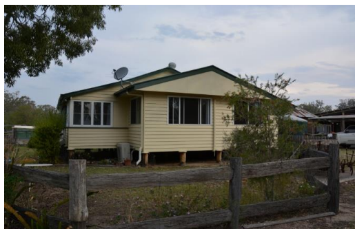
Figure 191. The south-west elevation of the caretaker's cottage, showing the contemporary extension in the foreground.
