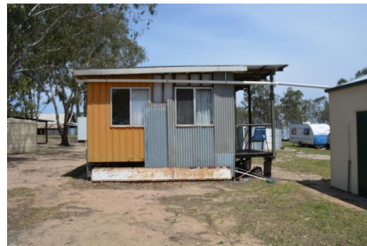
Figure 218. The north-eastern elevation of the archives building.
