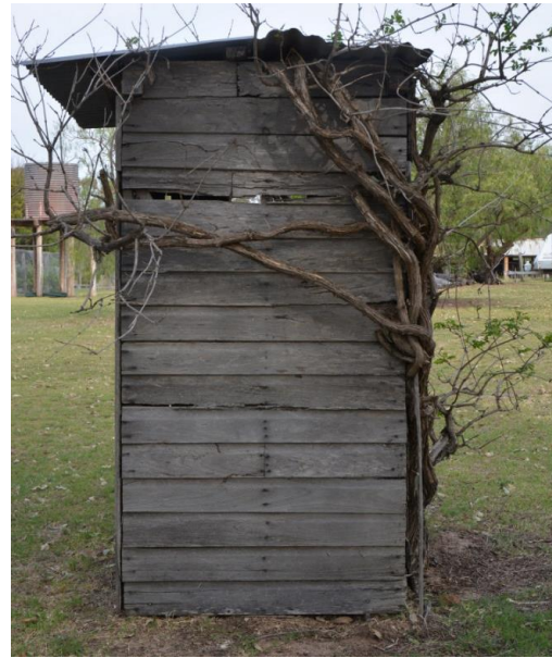
Figure 170. The north-west elevation of the outhouse, showing the extent of the tree growth around the structure.
