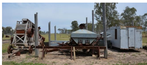
Figure 251. The north-eastern side of the former machinery shed, which now contains a display of machinery pieces within a series of timber posts.
