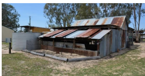
Figure 246. The north-western elevation of the camp kitchen.
