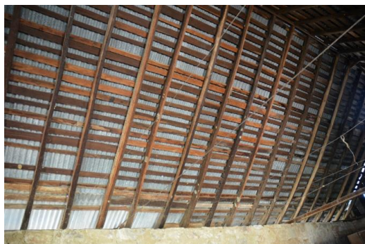
Figure 142. Detail view of the stone store's exposed internal roof structure.
