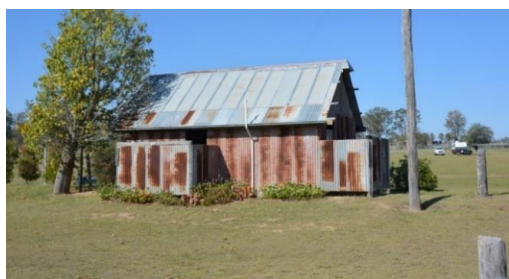
Figure 262. The north-east elevation of the toilet block located a short distance to the south-east of the stone store building.
