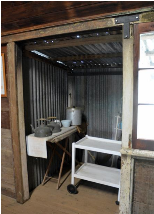
Figure 124. The kitchen stove recess, lined with corrugated iron contained with a skillion-roof addition.
