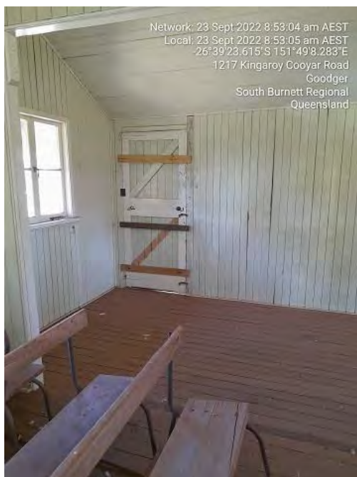
Rear door secured closed.
