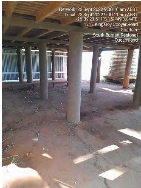
Typical timber stumps.
