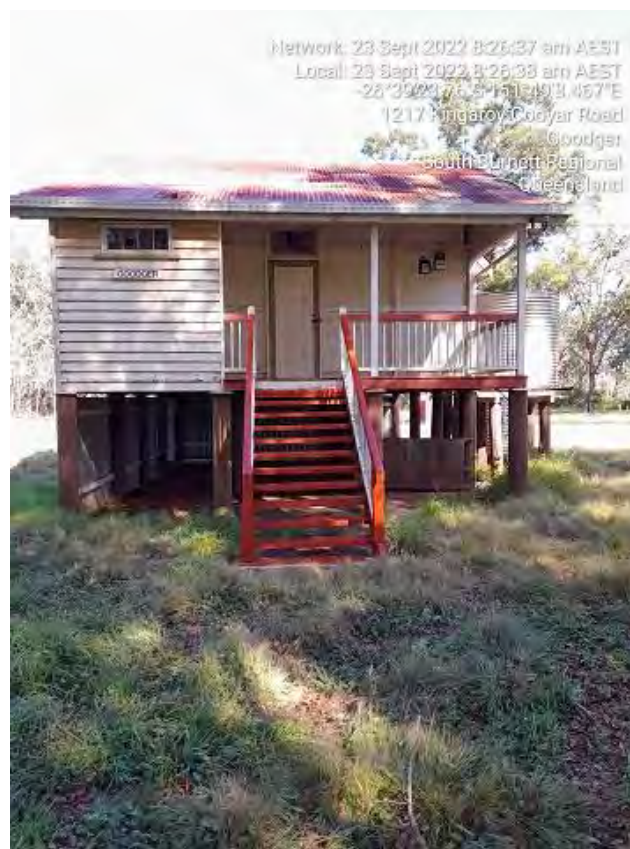
Front of Building
