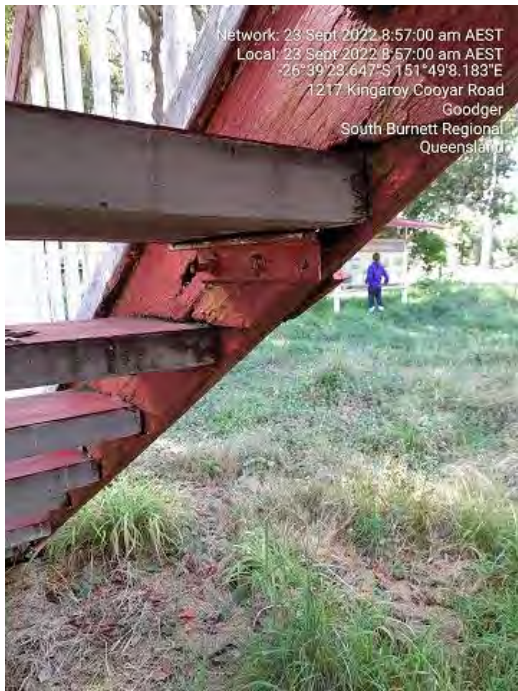
Front Stairs – Strings and Treads
