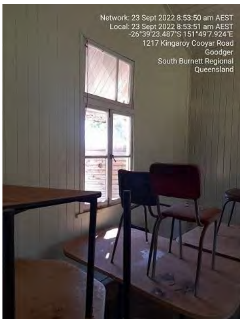
Internal wall with termite damage repaired.
