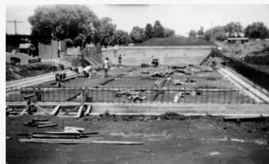
Figure 5: Construction of the pool in 1952 (Source: South Burnett Regional Council)
