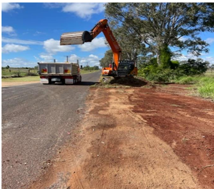
Photo: Siefert St – Drainage Works underway
