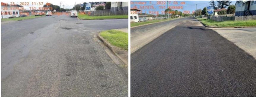
Photo: King Street before and after repair works
