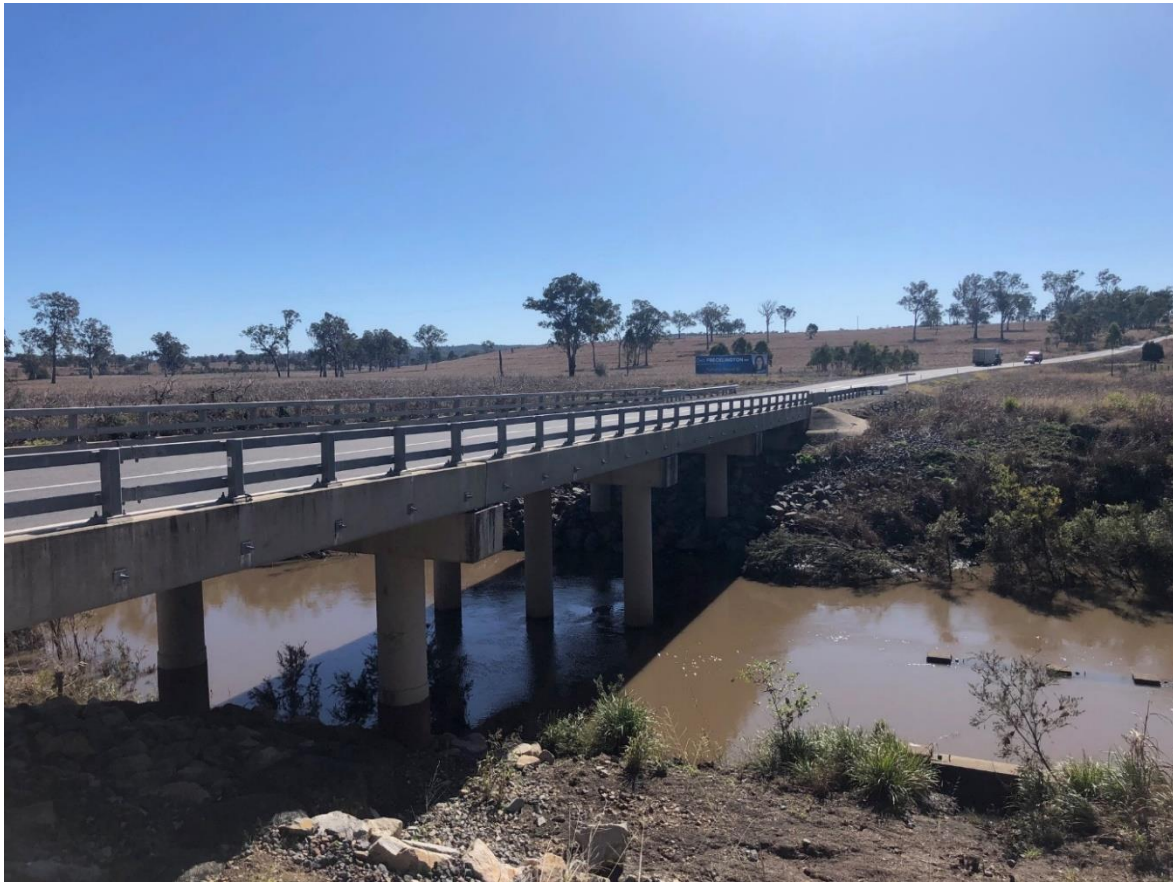
Figure 5: Burnett Highway Bridge Crossing - Barambah Creek
