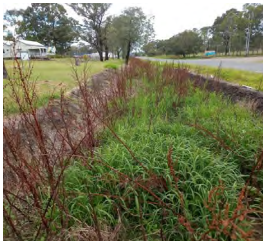
Overgrown and silted drain along Murgon Gayndah Road between Somerville Street and Gesslers Road
