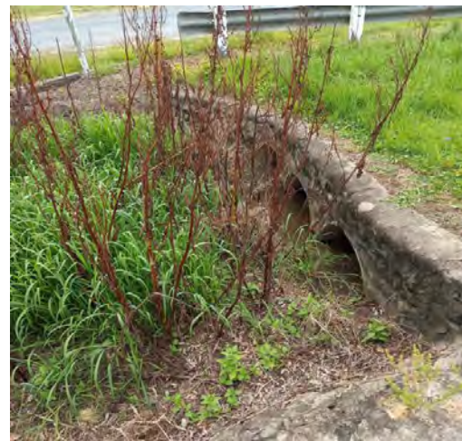
Overgrown and silted drain along Murgon Gayndah Road between Somerville Street and Gesslers Road
