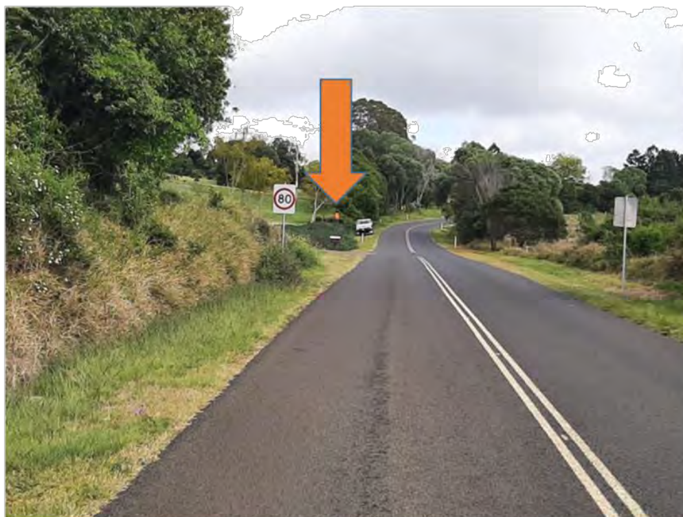
Figure 3 – Sight Distance of 130 metres to proposed access from the east 2x zoom for clarity
