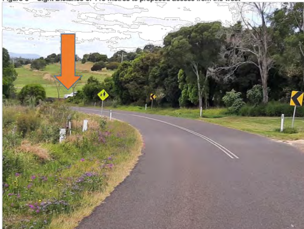
Figure 6 – Sight Distance of 115 metres to proposed access from the west 2x zoom for clarity
