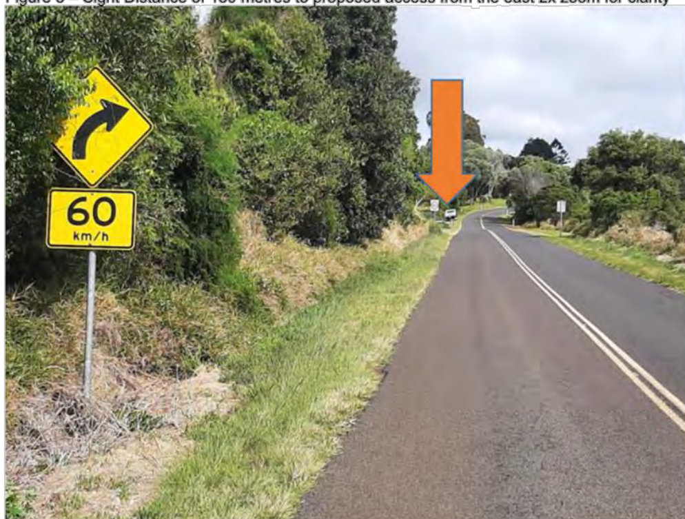
Figure 4 – Sight Distance of 180 metres to proposed access from the east 2x zoom for clarity
