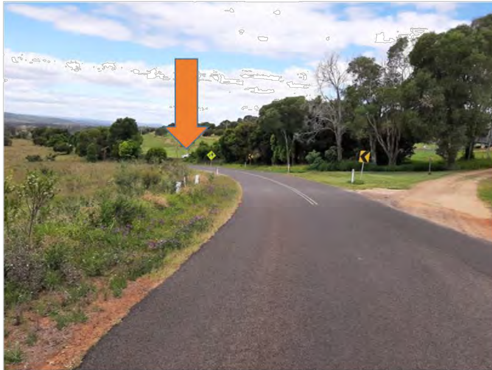
Figure 5 – Sight Distance of 115 metres to proposed access from the west
