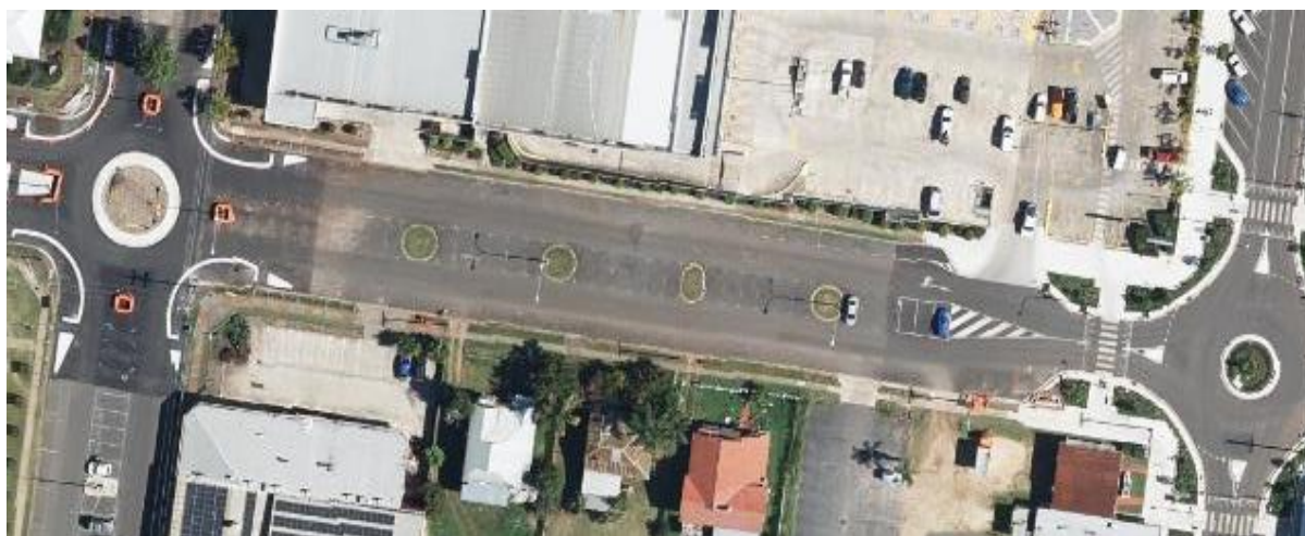
Figure One: Aerial view of grassed medians located on Glendon Street, Kingaroy (Alford St – Markwell St)
