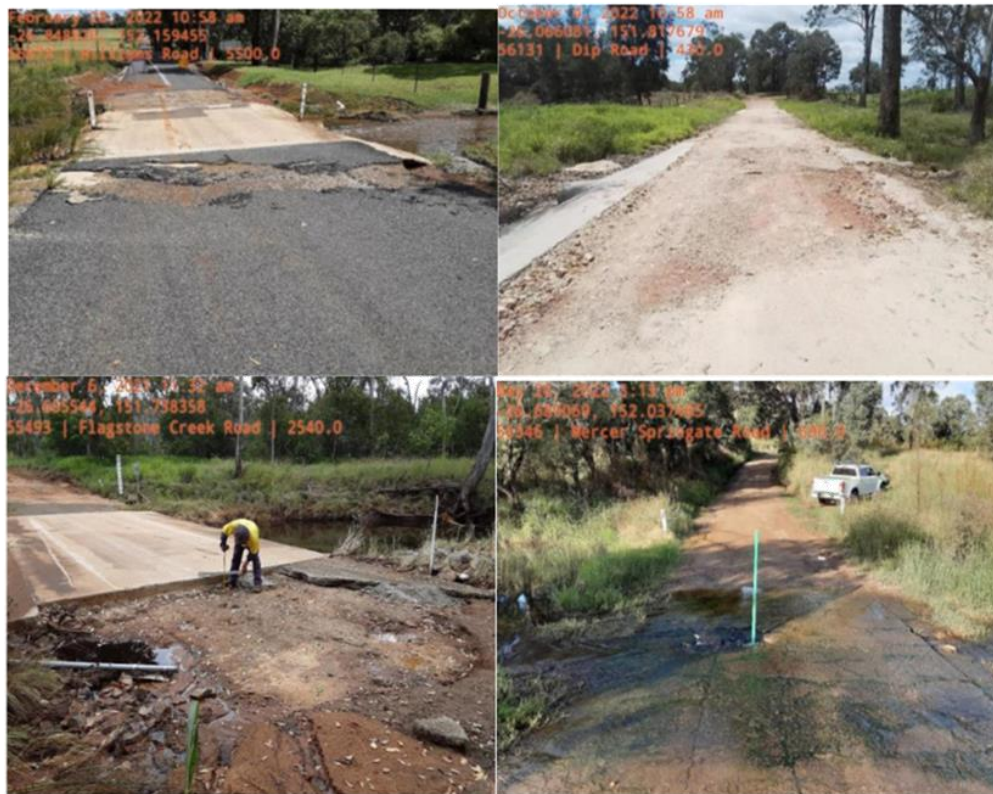
Betterment Location Photographs: Williams, Dip, Flagstone Creek & Mercer Springgate Roads
