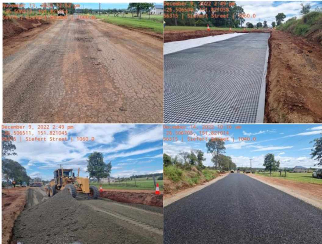
Photo: Siefert St, Crawford – REPA & Holding Works
