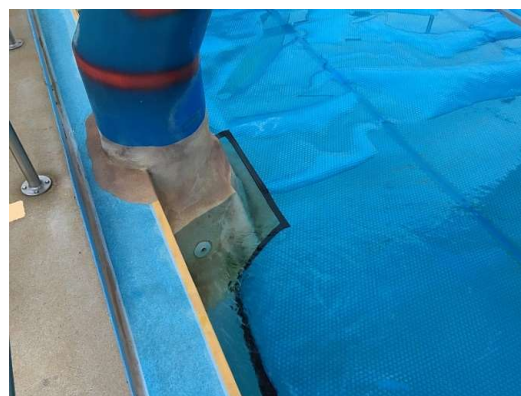
Rock Styled Inserts to Conceal Pipework.
