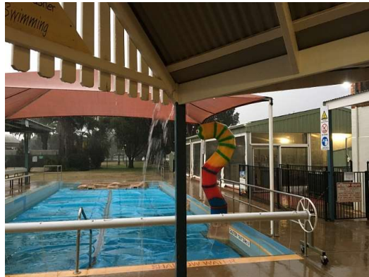
Features added to existing Wading Pool.
