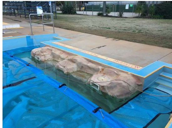
Skimmer Boxes added to existing Wading Pool.
