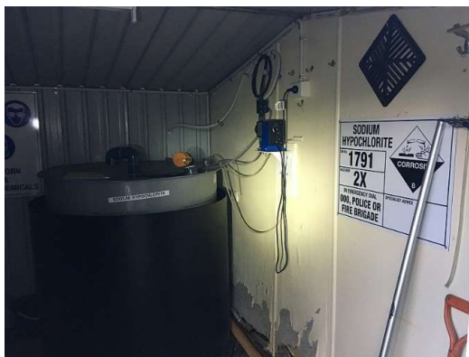
Sodium Hypochlorite Storage Tank and Bund.
