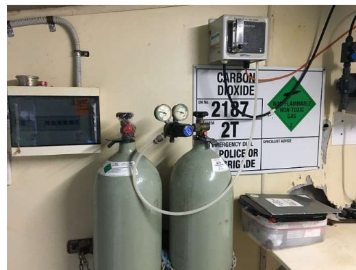
Pool Water Chemistry Dosing.
