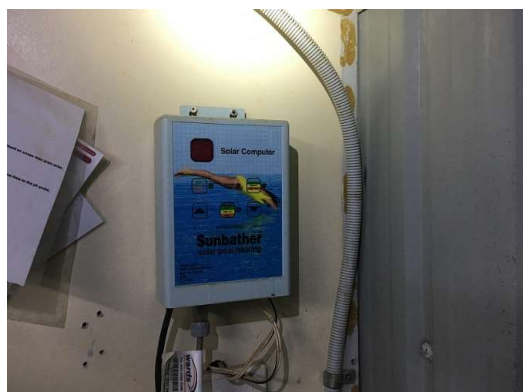
Existing Solar Controller.
