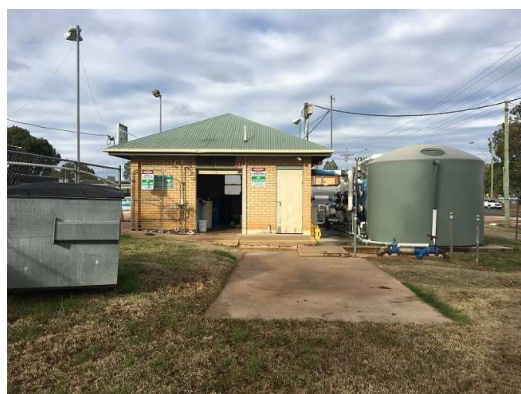
Truck Loading with Pool Plantroom Beyond.
