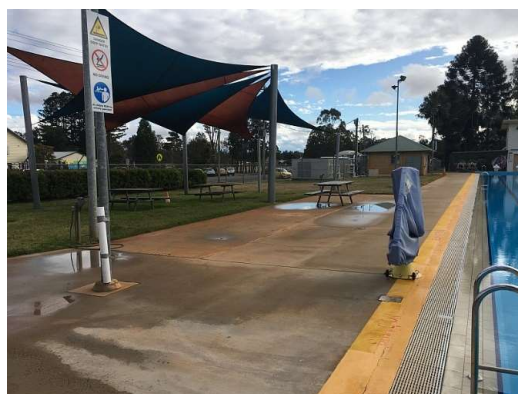
Typical Pool Concourse Finish with Pool Hoist.
