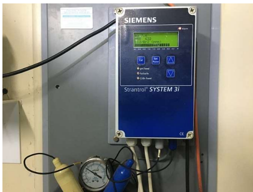
Pool Water Chemistry Instrument.
