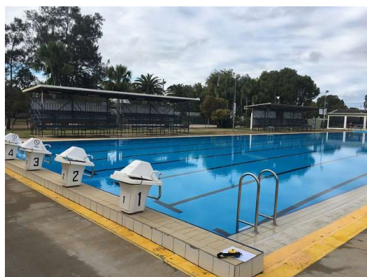
Existing 50m Pool.
