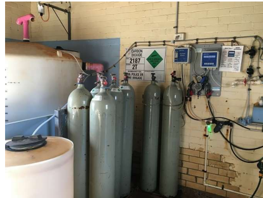
Pool Water Chemistry Dosing.
