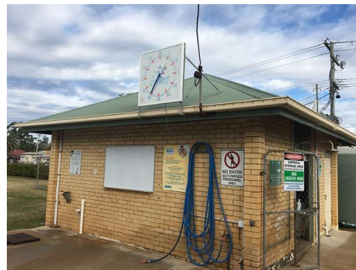
Signage and Pool Plantroom.
