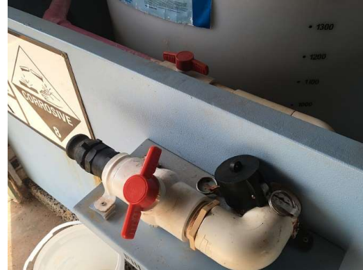
Tank Fill Point with Compact Ball Valve.
