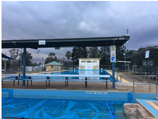
Typical Pool Signage at Concourse and Pool.
