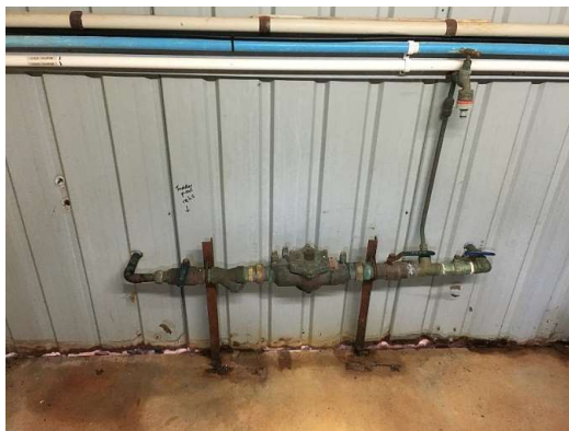
Water Supply to Pool.
