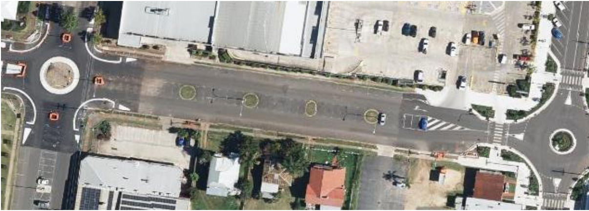
Figure One: Aerial view of Glendon Street, Kingaroy (Alford St – Markwell St) Ch250 to Ch360
