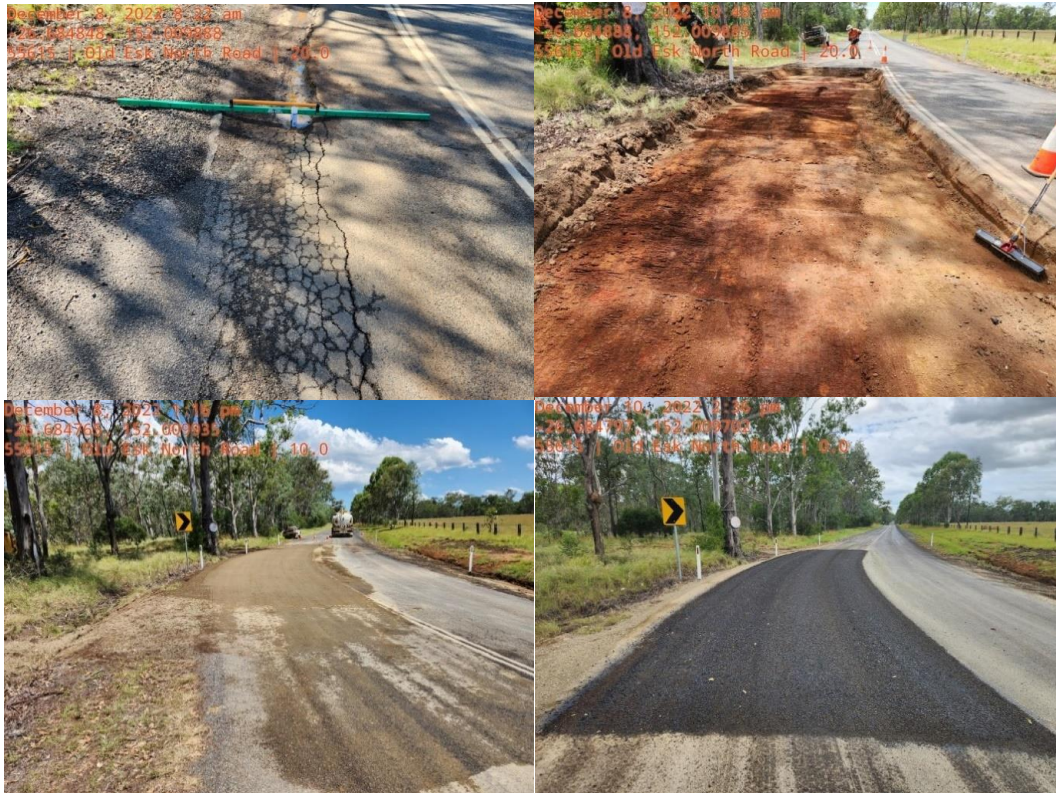
Photo: Old Esk North Road, South East Nanango – REPA & Holding Works
