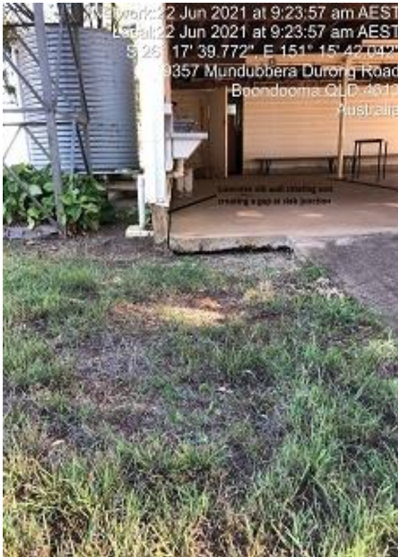
Nib wall rotated and moved.
