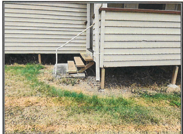
Down pipes discharging to ground surface adjacent foundations
