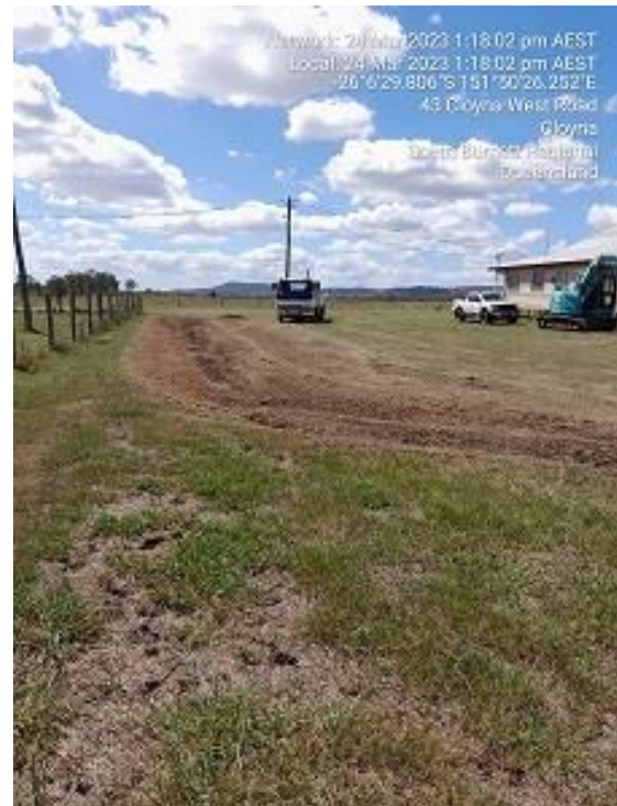
Site drainage works.
