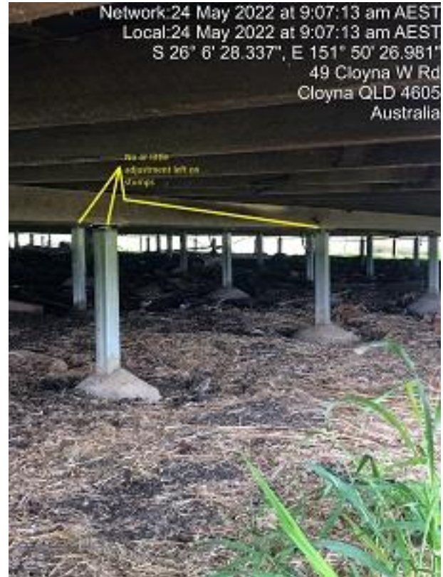
No adjustment left in stump tops.
