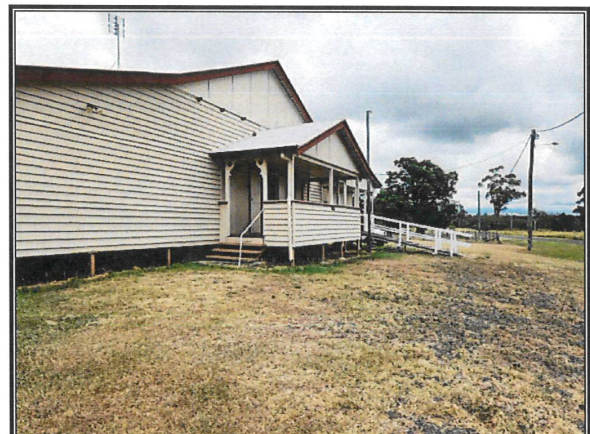
Good site drainage to northern side of hall
