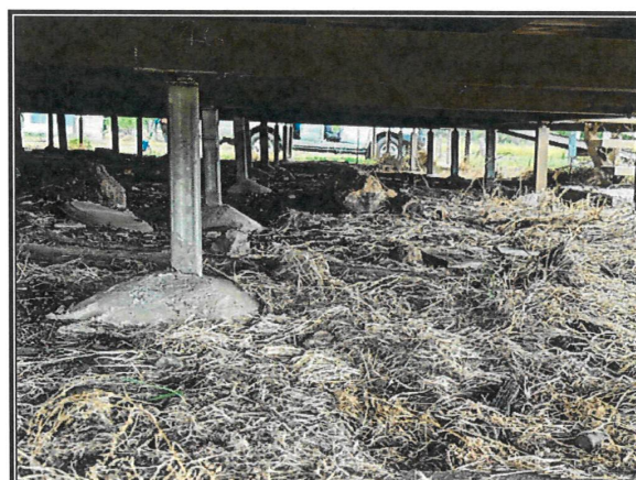
SHS subfloor posts have been cut and re-welded to allow for further adjustment
