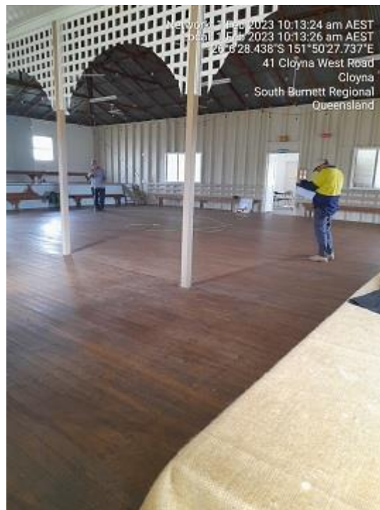
Measuring floor deflection.
