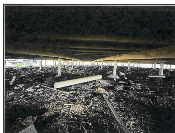
Visual upward bow of floor bearers
