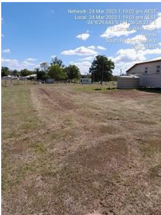
Site drainage works.
