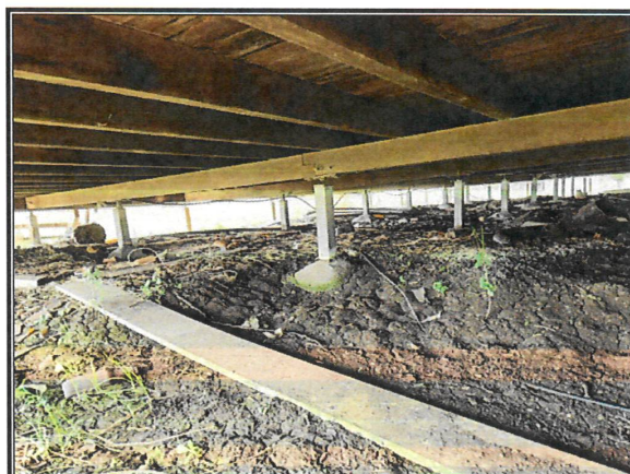
Rusting of bases of SHS subfloor posts
