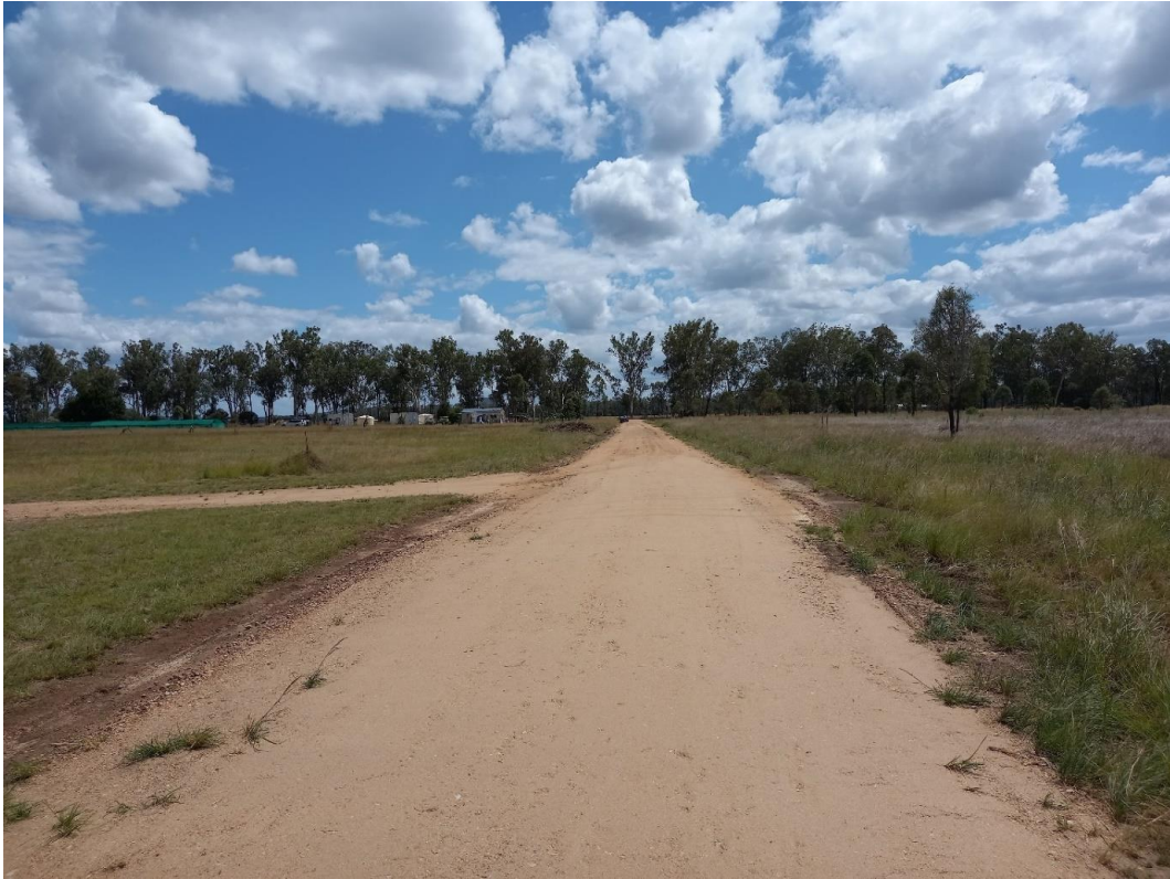
Figure 2: New road looking South towards Mondure Wheatlands Road (18/01/2023)
