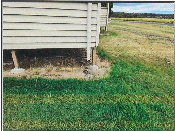
Down pipes discharging to ground surface adjacent foundations
