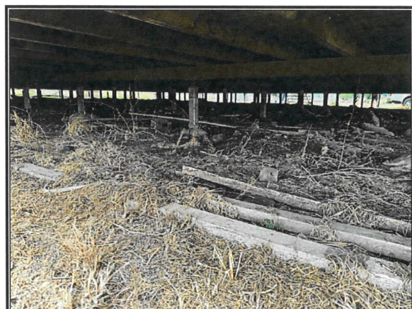
SHS subfloor posts have been cut and re-welded to allow for further adjustment
