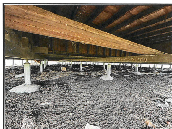
Visual upward bow of floor bearers
