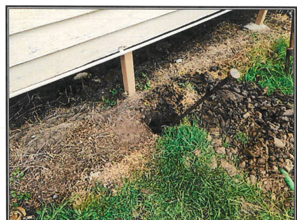
Inspection of existing foundations
