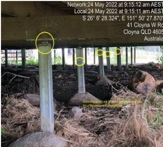
Cut stumps and no adjustment.
