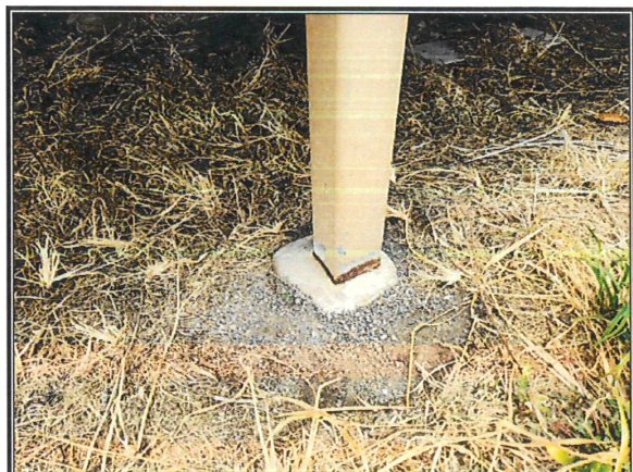
Rusting of bases of SHS subfloor posts
