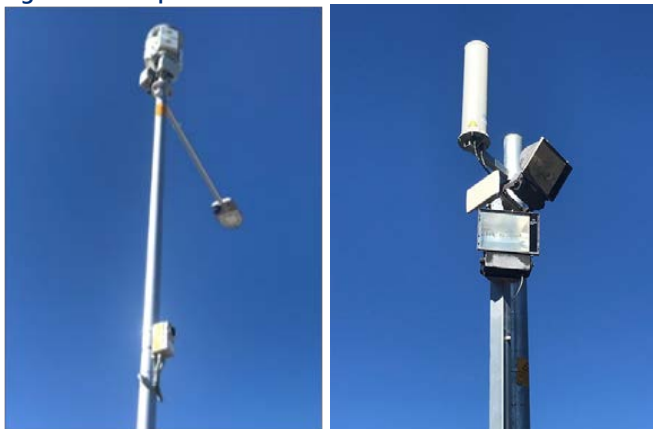
Figure 5: Example of co-located facilities
