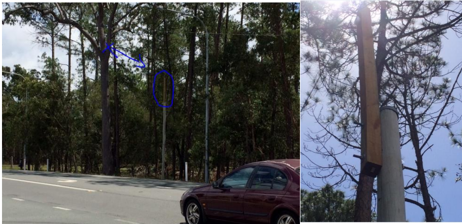
Figure C: Telecommunications overhead line installed by a telecommunications contractor in a tree.
