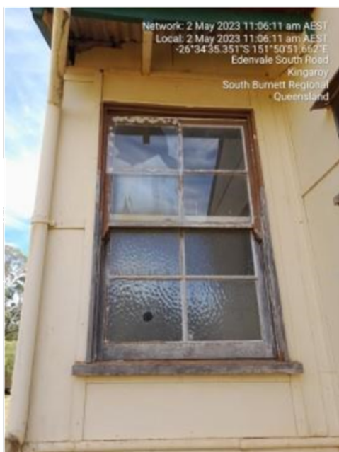
Typical timber double hung window.
