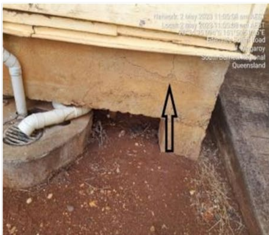
Cracked slab.
