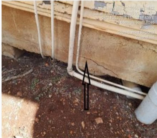
Cracked slab.
