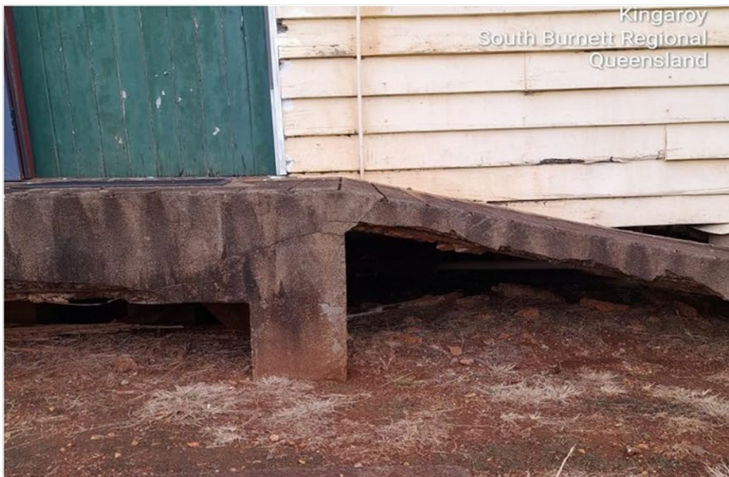
Ramp to Eastern Side
