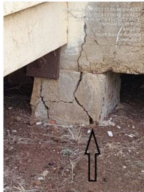
Slab/stump deterioration.
