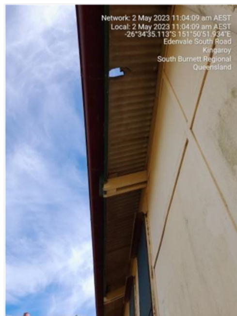
Damaged roof.
