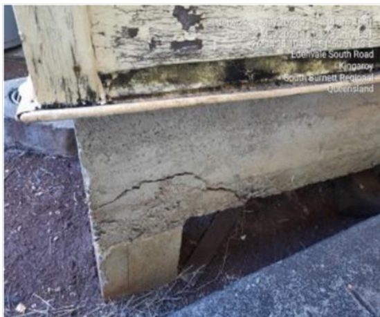
Slab damage.
