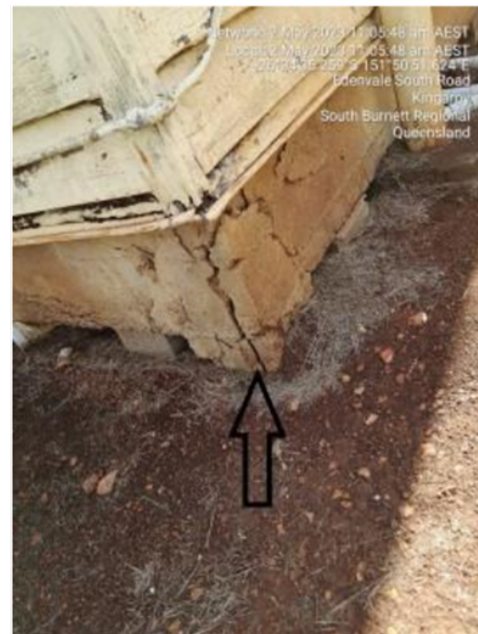
Slab damage.
