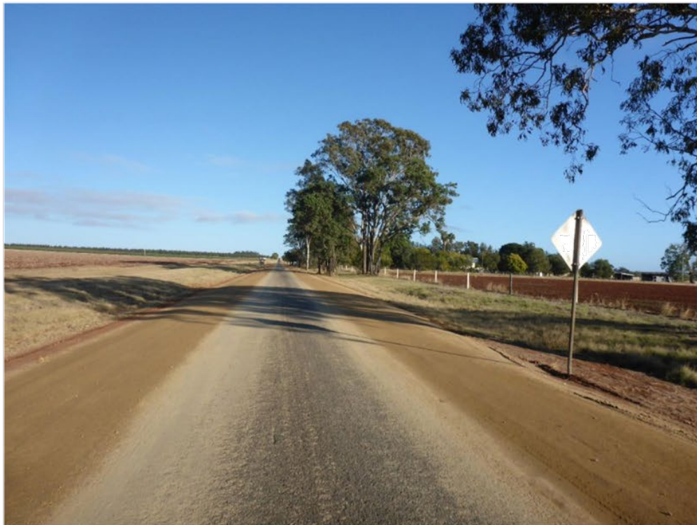
Shoulder Resheeting – Reedy Creek Road, Benair
