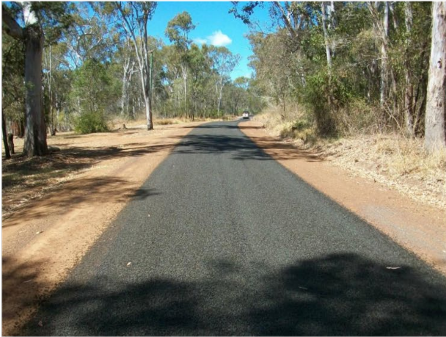
Bitumen Resealing - Old Esk Road, Taromeo
