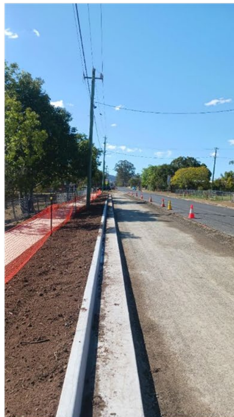
Parking Improvements - Gore Street, Murgon
