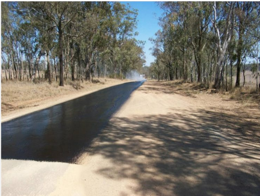
Bitumen Resealing – Runnymede Road , Runnymede
