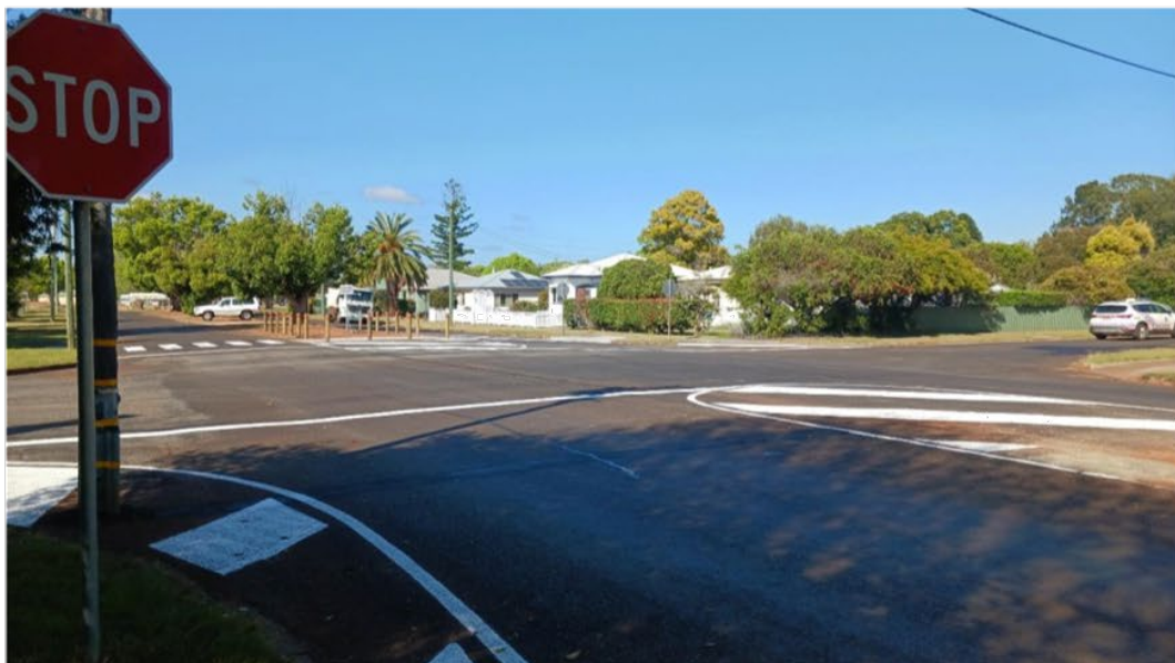
Pedestrian Crossing Improvements – William Street, Kingaroy
