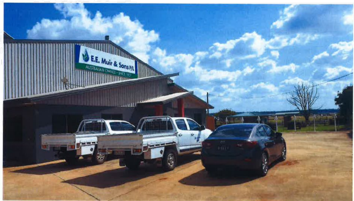
Photograph 2 View to the west of the front carpark and retail store
