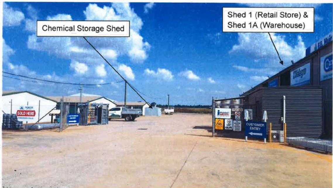
Photograph 1 View to the south of the site entrance
