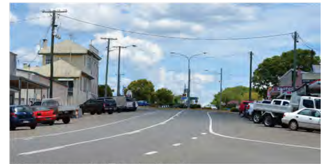
Existing view approaching the town from the north
