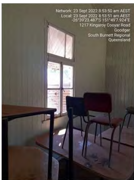
Internal wall with termite damage repaired.
