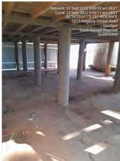
Typical timber stumps.
