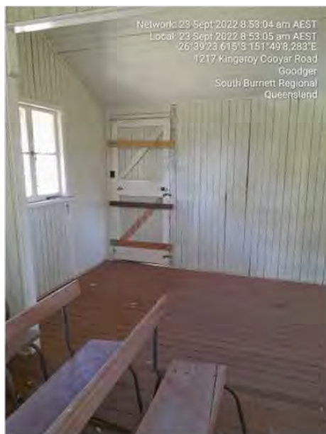
Rear door secured closed.
