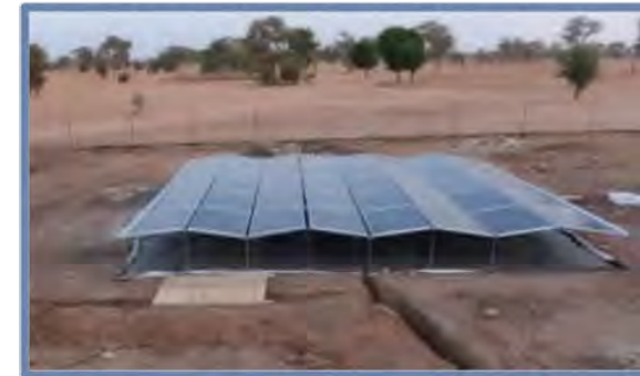
Kalom, Senegal, 20kWp (2016)
