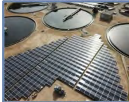
Hoensbroek, Netherlands, 2MWp (2020)
