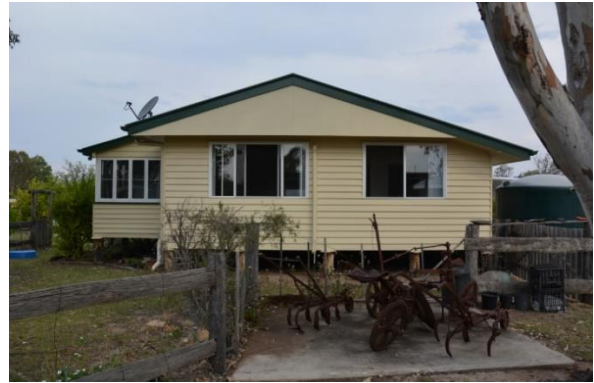
Figure 192. The south-west elevation of the caretaker's cottage.
