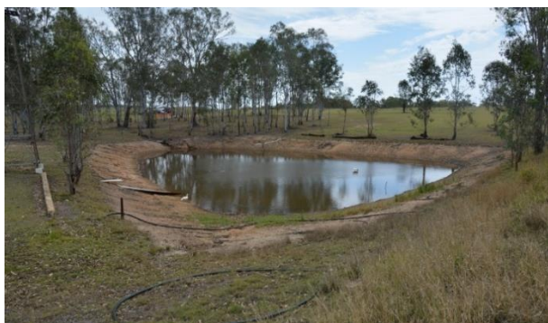
Figure 268. View facing north-west of the dam located on the Boondooma Homestead property.
