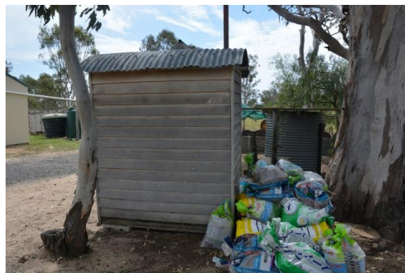
Figure 259. One of the timber outhouses used for storage.
