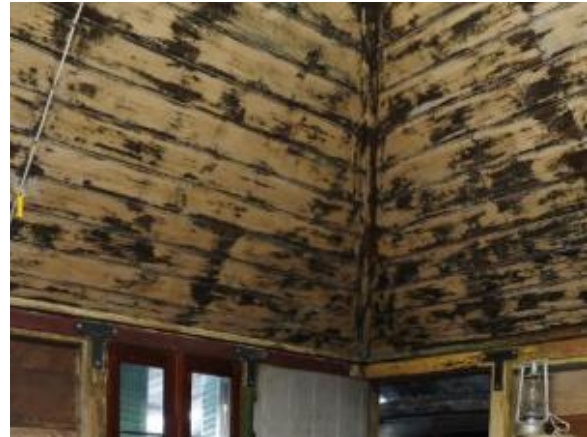
Figure 127. Detail of the ceiling of the detached kitchen, lined on the rake with unpainted, horizontally-fixed beaded boards.
