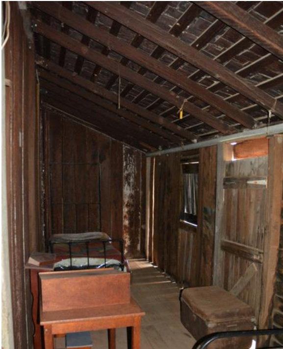
Figure 118. Interior of Bedroom 3, showing the surviving roof shingles fixed under the roof sheet.
