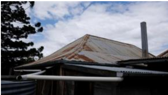
Figure 86. View facing north-east showing the 'broken back' roof profile of the main homestead, and the skillion-roof of one of the small extensions.
