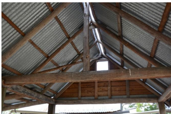
Figure 159. Interior view of the reconstructed timber roof framing built using traditional bush carpentry construction.
