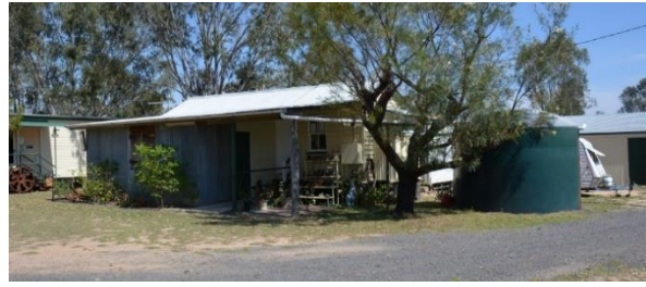
Figure 214. View facing west of the administration building, showing the large water tank adjacent at the right and behind that, the demountable amenities block (not visible).
