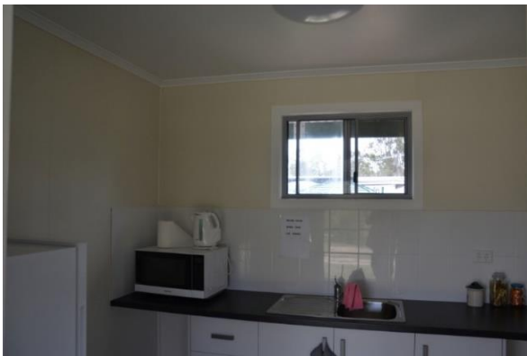
Figure 242. Interior of the kitchenette in the accommodation building.
