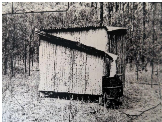
Figure 31. The structure known as the boundary rider's hut photographed in situ prior to 1999 on the property known as Delger . Source: Boondooma Museum & Heritage Association (2021) 55
