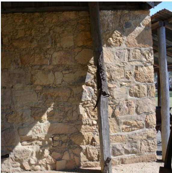
Figure 135. Typical example of the central core, constructed of large sections of stone arranged roughly in courses, between which smaller pieces have been inserted.
