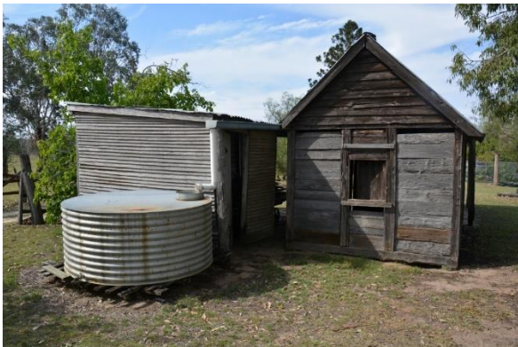
Figure 171. The rear south-west elevation of the postal receiving office, showing the adjacent carport skillion-roof extension and water tank.
