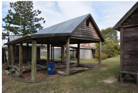
Figure 158. View facing north-east of the incomplete reconstruction of the detached c.1870s 'dining room' structure, or possibly an earlier dwelling.
