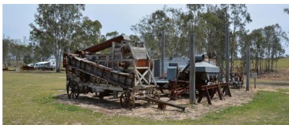
Figure 250. The south-eastern corner of the former machinery shed, with contemporary timber posts re-erected in recent decades to show where the structure once stood.
