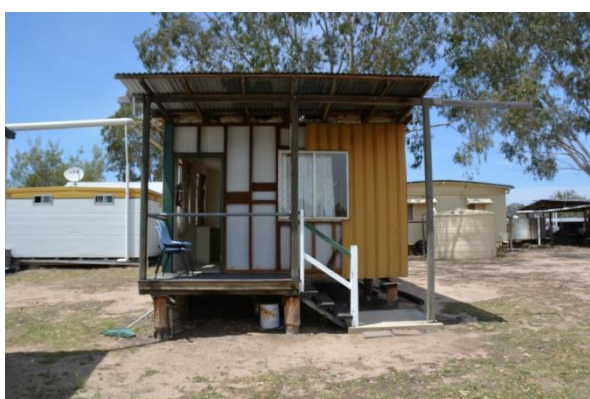
Figure 219. The main north-western elevation of the archives building, showing the external timber stair and landing.
