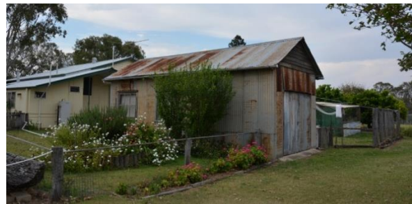
Figure 196. View facing north of the caretaker's store, with the caretaker's cottage visible adjacent in the left background.
