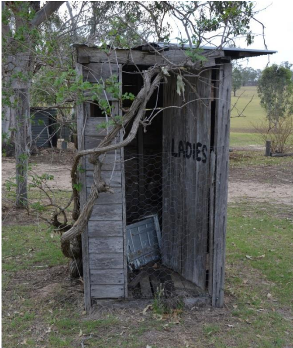
Figure 169. The south-east elevation of the outhouse.
