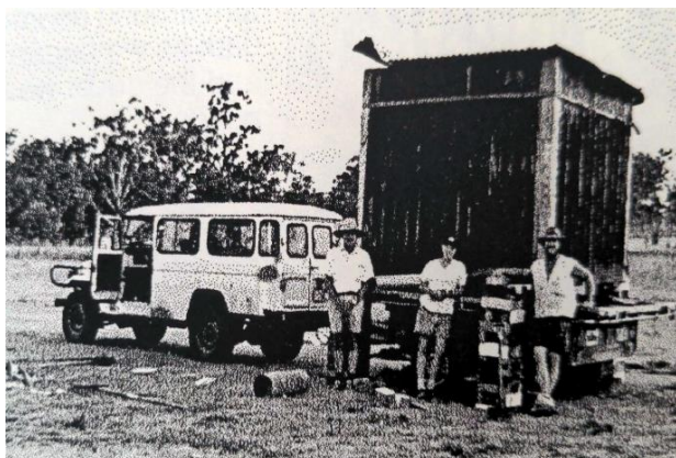
Figure 30. Lionel, Helen, and Phill pose in front of the structure known as the boundary rider's hut following its relocation to Boondooma, where it was re-stumped. Source: Boondooma Museum & Heritage Association (2021) 54
