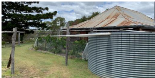
Figure 83. The north-west elevation of the main homestead.
