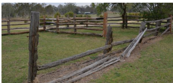
Figure 182. View facing south-west from showing the combination of dilapidated timber posts and rails comprising the former stockyards and recently reinstated erect sections.
