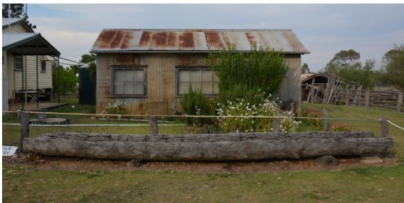
Figure 195. The south-west elevation of the caretaker's store.
