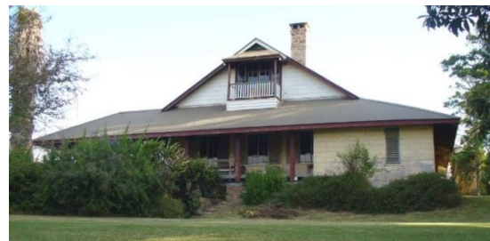
Figure 53. Top and Bottom: Cressbrook Homestead in 2005 and 2007. Source: Queensland Government (2016c).
