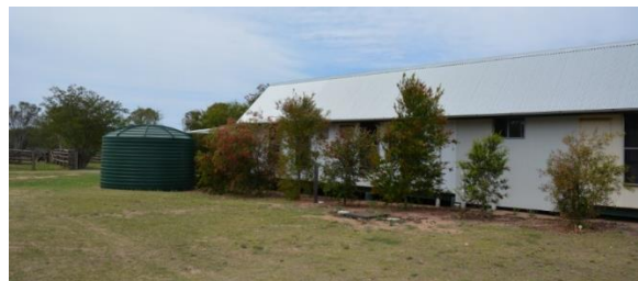
Figure 241. The north-west elevation of the accommodation building.
