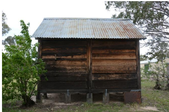
Figure 166. The north-east elevation of the cool house.
