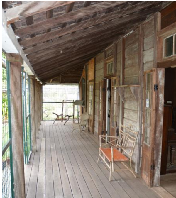
Figure 91. View along the front verandah of the main homestead, showing the eastern end of the verandah.
