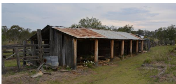
Figure 181. The north-west elevation of the milk bails structure. Note the rough-sawn timber slabs, fitted vertically, that partially enclose the structure at this end and the timber posts supporting the structure.
