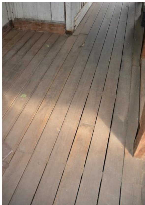
Figure 101. Example of the typical verandah floorboards on the homestead's verandahs, which is lined with shot-edge boards.
