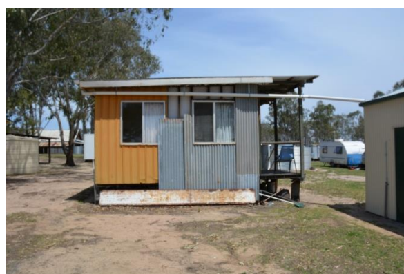
Figure 218. The north-eastern elevation of the archives building.
