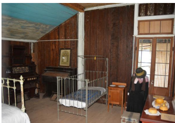
Figure 108. Interior of Bedroom 1, the main bedroom in the homestead. Note the low-pitched ceiling, partly painted, falling from the beam that may once have contained a wall. Some of the timber framing elements are also painted.
