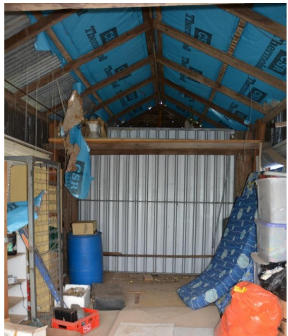
Figure 198. Typical interior of the caretaker's store.
