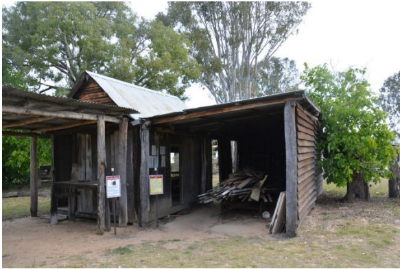
Figure 175. View facing south-west of the postal receiving office showing the adjoining carport extension.
