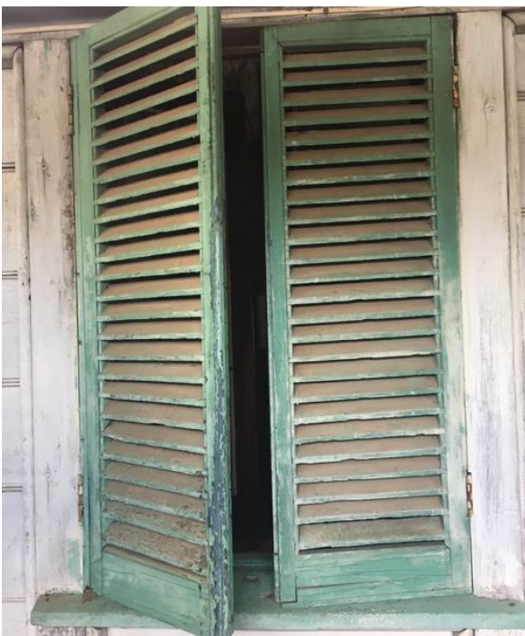
Figure 92. Example of the homestead's timber-framed windows with fixed-louvre shutters.
