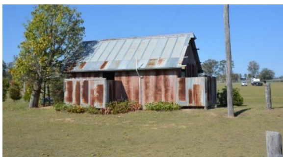
Figure 262. The north-east elevation of the toilet block located a short distance to the south-east of the stone store building.
