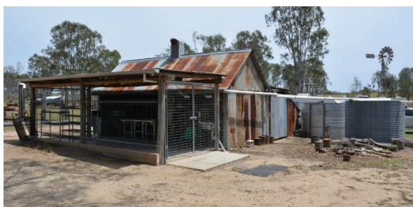
Figure 247. The south-eastern elevation of the camp kitchen.
