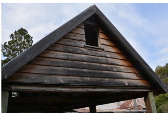
Figure 161. Detail of the timber gable infill.
