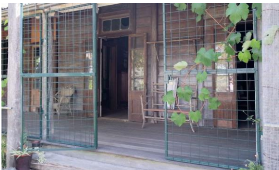
Figure 88. The front verandah of the main homestead, showing the modern, powder-coat steel, grid-mesh screening that encloses the verandah for security purposes.
