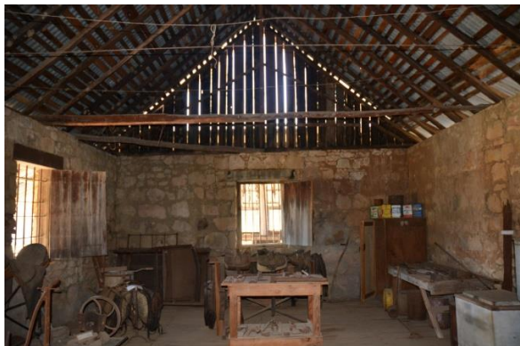
Figure 143. Interior of south-east end of the stone store. Note the two windows with vertical iron bars and timber shutters.
