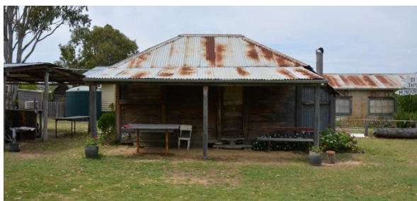
Figure 199. The main south-west elevation of Brownie’s hut.
