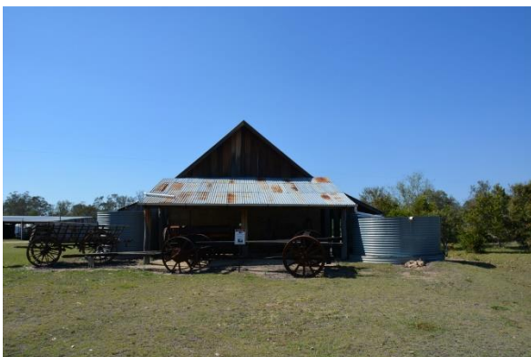
Figure 133. View of the north-west elevation of the stone store building, noting the two water tanks attached either side of the structure.
