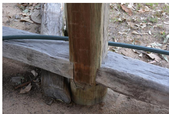
Figure 162. Detail of the intersection of a column and bearer reconstructed using traditional bush carpentry techniques.
