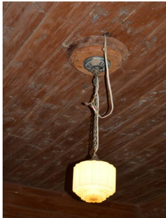
Figure 106. Detail of the single pendant light fitted in the central dining room.
