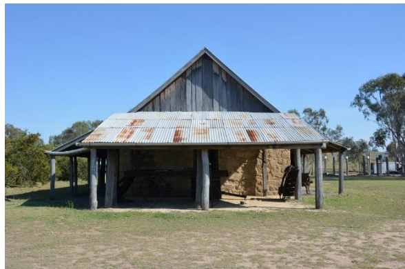
Figure 132. The south-east elevation of the stone store building, where the lean-to verandah addition is utilised for the display of a historical wagon.
