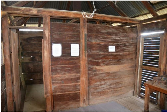
Figure 203. Interior of Brownie's hut showing the dividing wall between the two internal spaces.
