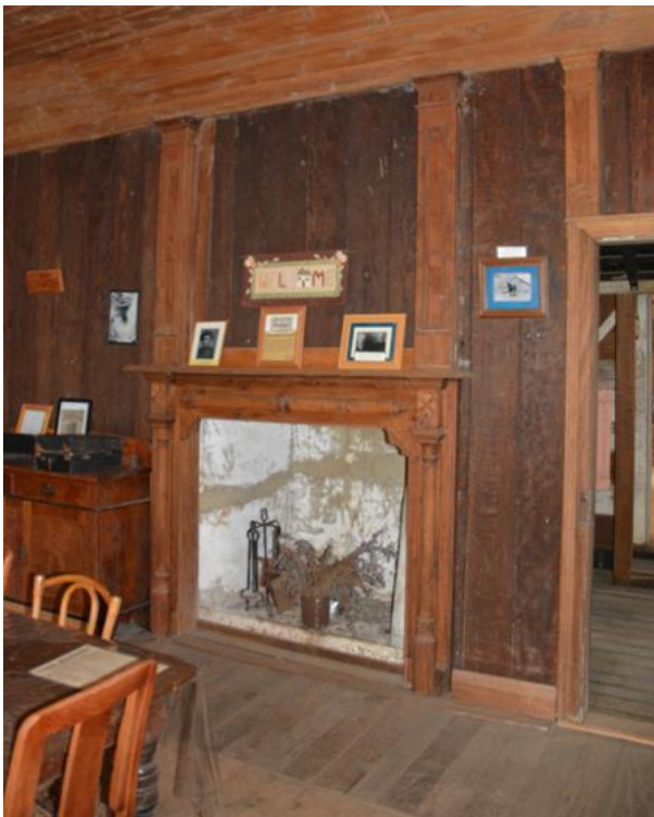
Figure 105. The dining room fireplace and timber mantelpiece, showing the fine timber joinery work.
