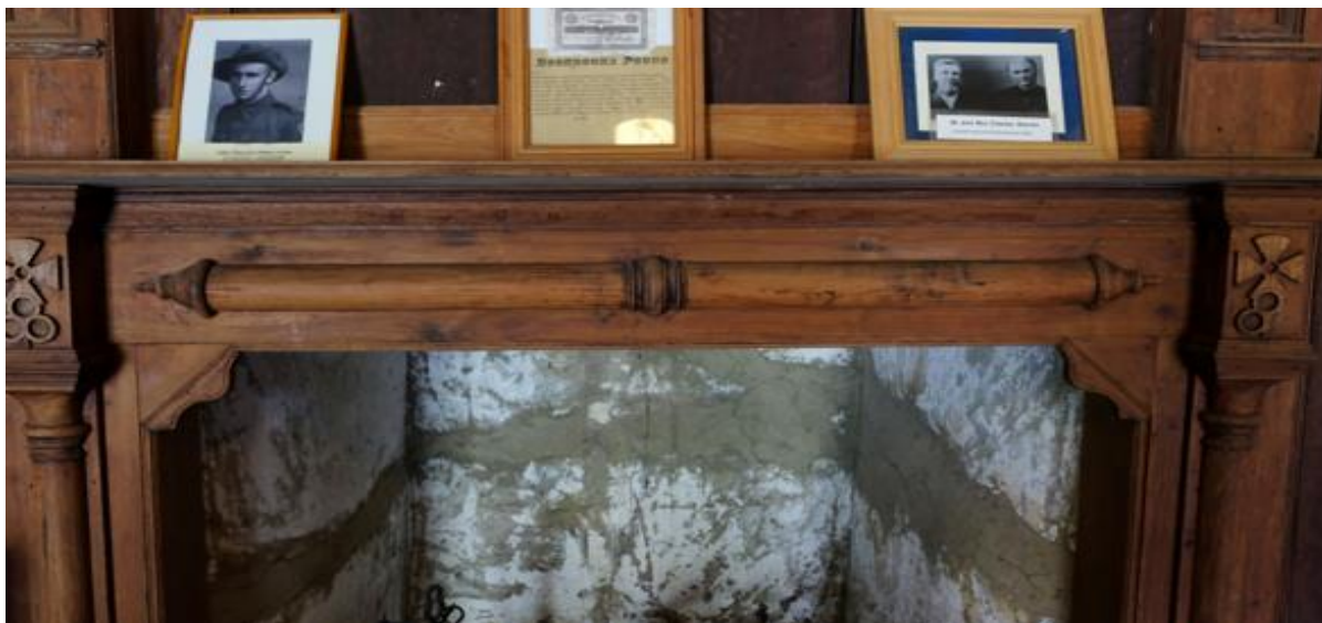
Figure 107. Detail of the timber mantelpiece of the dining room fireplace in the main homestead. Note the finely-detailed timber joinery and mouldings. The early shellack and wax finish of the mantelpiece has been removed.
