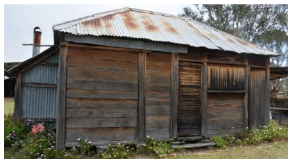
Figure 202. The north-east elevation of Brownie’s hut. Note the wide timber weatherboard slabs, fitted horizontally.
