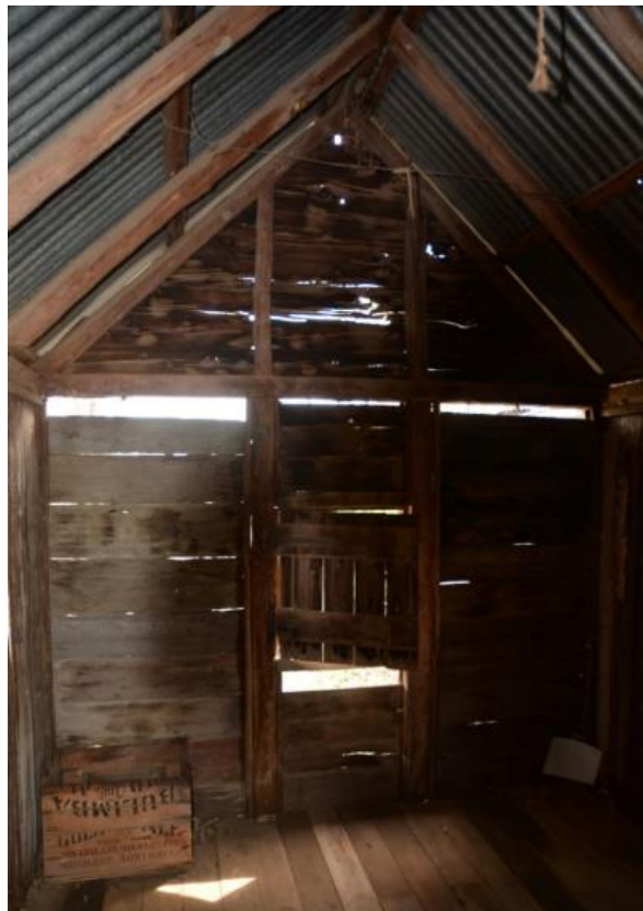
Figure 174. Interior of the postal receiving office with the timber casement window visible in the centre.
