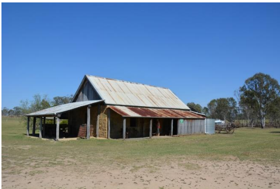
Figure 131. The north-east elevation of the stone store building.
