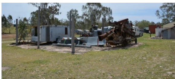
Figure 252. The south-western corner of former machinery shed.
