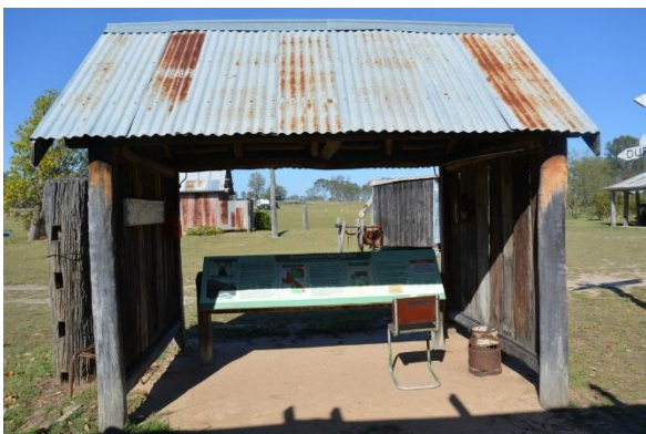
Figure 205. The north-east elevation of the DPI shelter.
