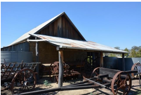
Figure 137. The verandah on the north-west elevation of the stone store building, used to display associated machinery pieces.
