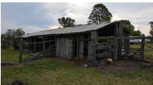
Figure 185. View facing west of the milking bails structure from within the stockyards.
