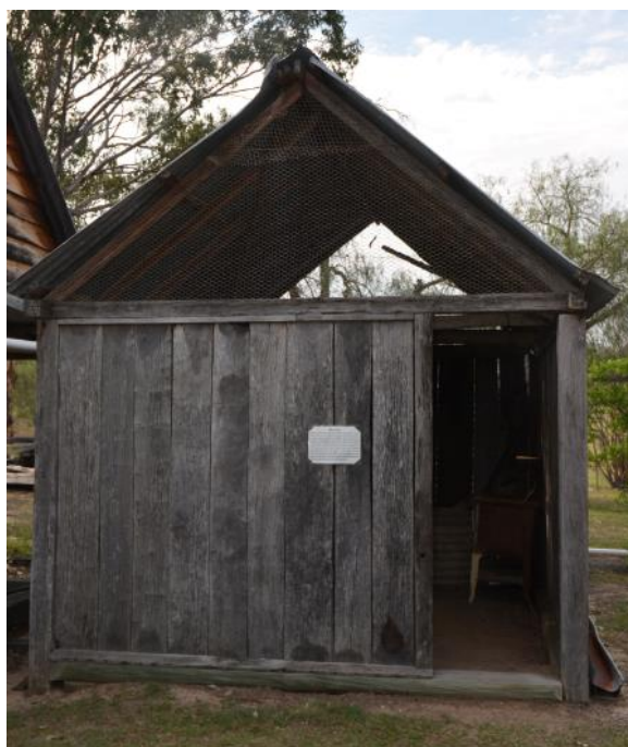
Figure 152. The main south-east elevation of the meat house.
