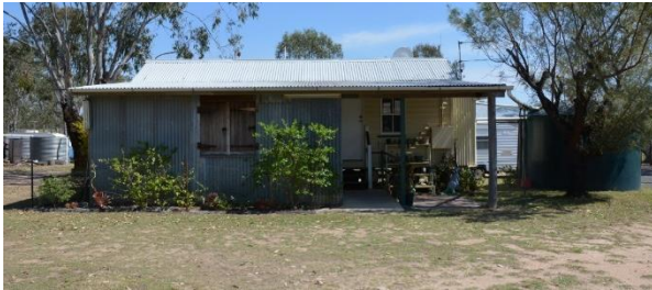
Figure 213. The main south-eastern elevation of the administration building.
