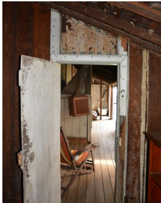
Figure 121. Interior view looking out from the study to the rear, semi-enclosed verandah.
