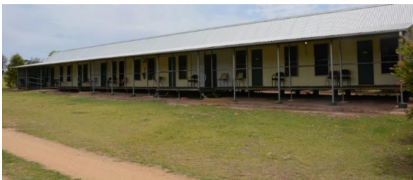
Figure 240. The south-east elevation of the accommodation building.
