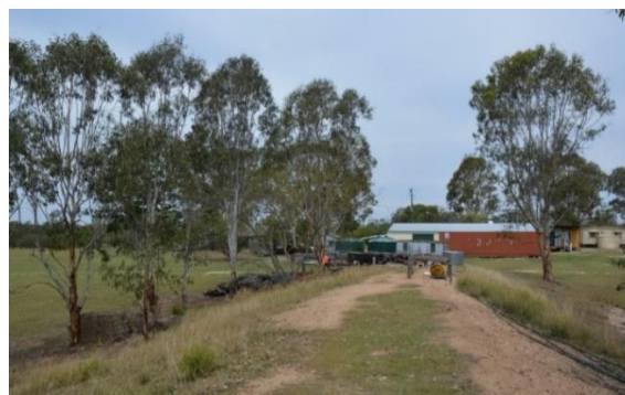
Figure 269. View facing south-east towards the main aspect of the Boondooma Homestead complex from atop the dam embankment.
