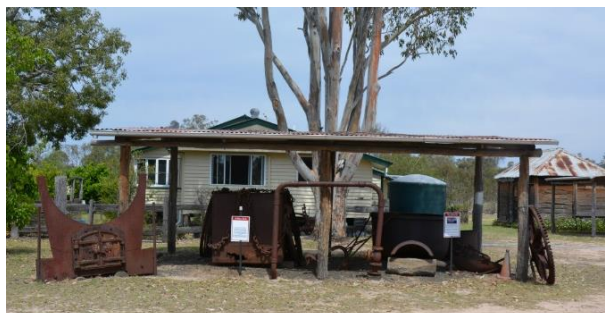
Figure 178. The north-west elevation of the tank display shelter, with the caretaker's cottage located behind.
