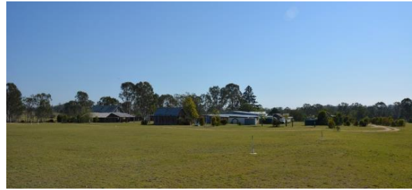
Figure 63. View from the open grassed area utilised for caravans and campers, facing north-east the main cluster of buildings and structures comprising the Boondooma Homestead complex.
