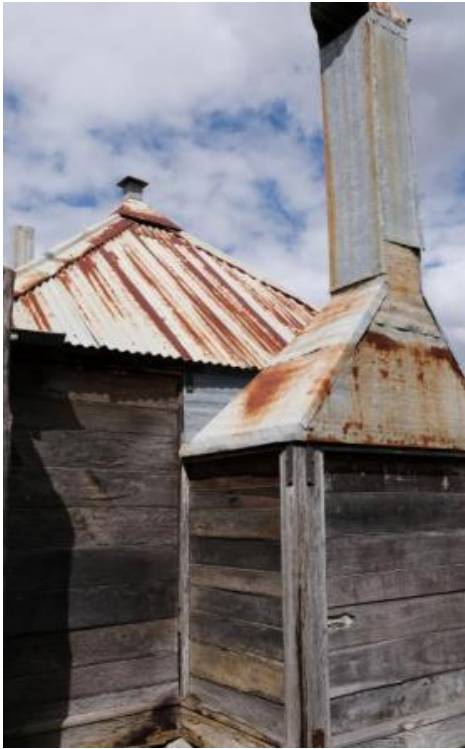
Figure 94. Rear of the detached kitchen on the south-west elevation of the main homestead, showing the pyramid roof profile and galvanised metal-clad chimney.
