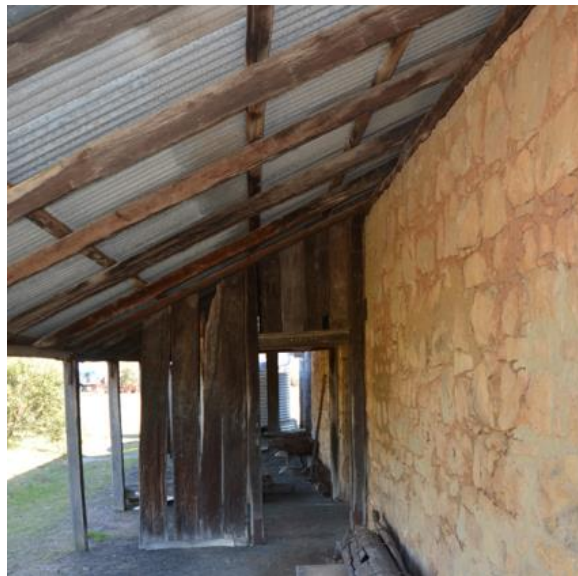
Figure 136. Example of the post-and-sapling frame construction of the lean-to verandah additions, which are reconstructions of earlier features.
