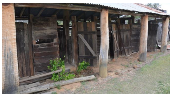
Figure 186. The timber slab doors that divide the milking bails structure internally to create individual stalls.
