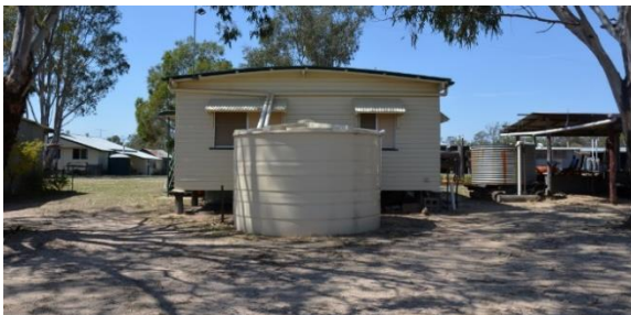
Figure 224. The south-western elevation of the museum building, showing the adjoining water tank.
