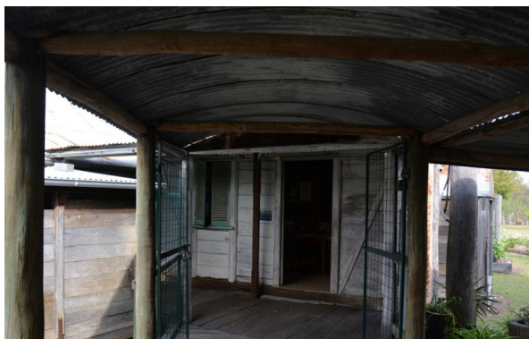
Figure 98. View from underneath the covered walkway facing towards the detached kitchen of the main homestead.
