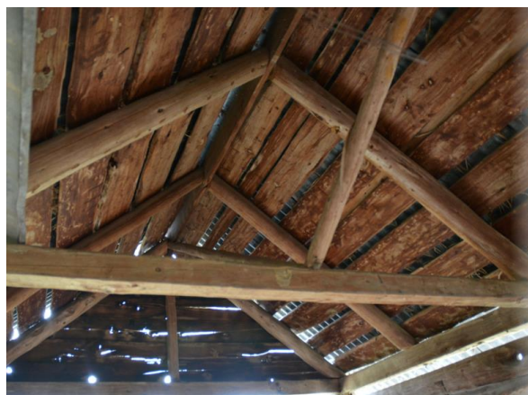
Figure 168. Interior of the cool house showing the gable roof form and horizontal timber slabs of Cypress pine.
