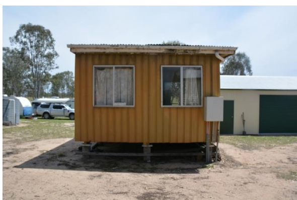
Figure 217. The north-eastern elevation of the archives building.
