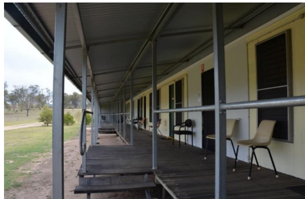
Figure 243. View facing south-west along the front verandah of the accommodation building, providing access to the individual bedrooms, kitchenette and bathroom.
