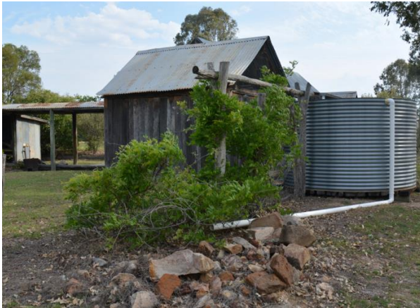
Figure 155. View facing south-west of the meat house, showing the adjacent water tank and timber trestle supporting the rainwater goods.
