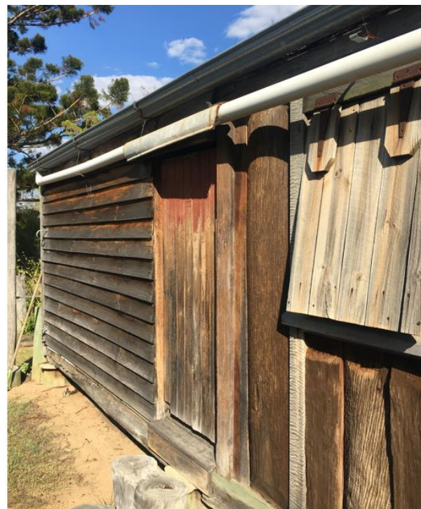
Figure 93. Detail of the external wall of the homestead's north-west elevation, illustrating the use of a variety of materials including unpainted weatherboards, fixed horizontally, and wide chamber boards, fitted vertically.
