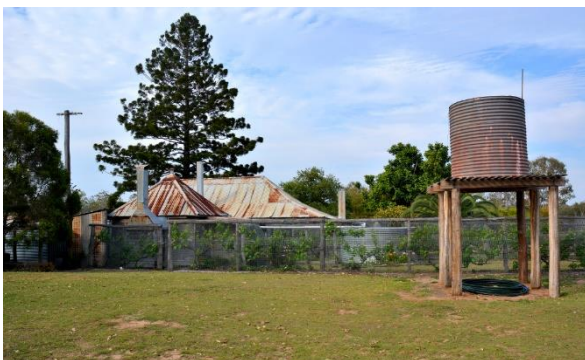
Figure 60. View facing east of the rear elevation of the main homestead from the open space between the cluster of other historical structures.
