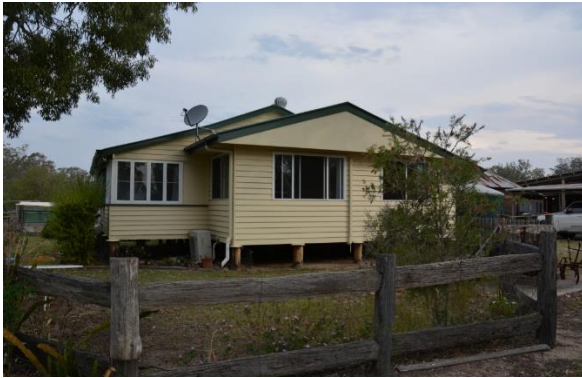
Figure 191. The south-west elevation of the caretaker's cottage, showing the contemporary extension in the foreground.
