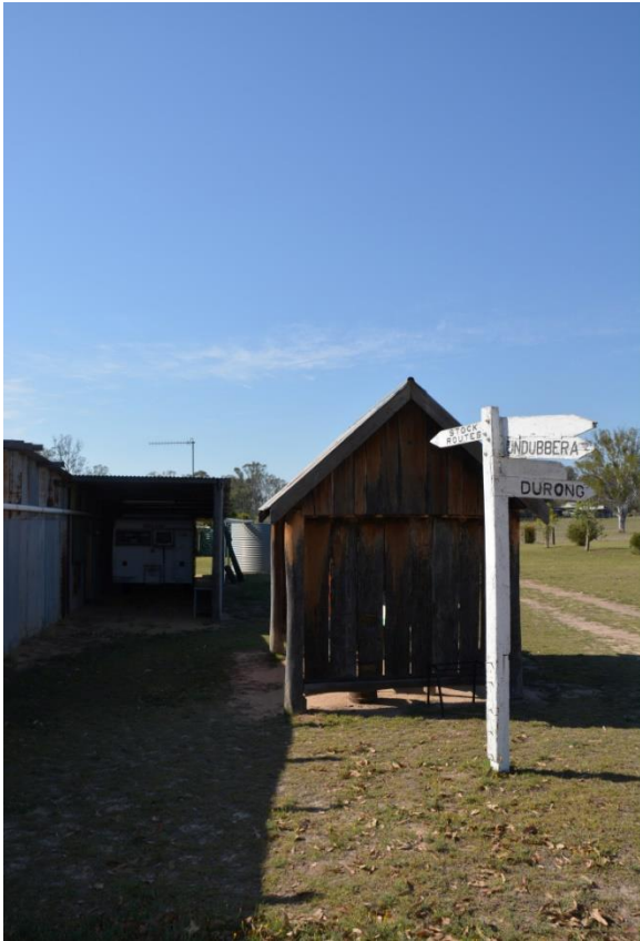
Figure 207. The north–western elevation of the DPI shelter, with the rear elevation of the ‘Big Top’ entertainment area structure adjacent at the left.
