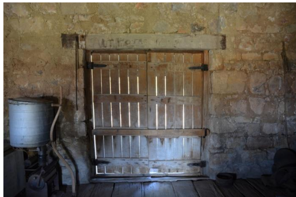
Figure 144. Detail of the timber double doors, which provide access to the stone store.
