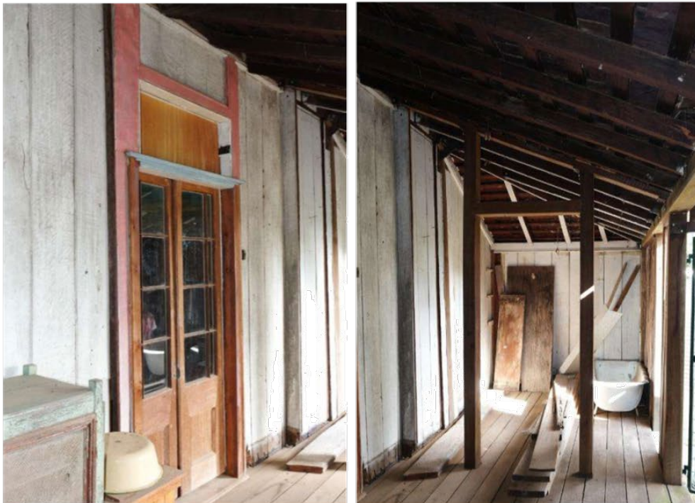
Figure 14. Left: The French doors from the main bedroom onto the rear verandah, noting the infilled fanlight. Right: View along the rear enclosed verandah area to the south-west.
