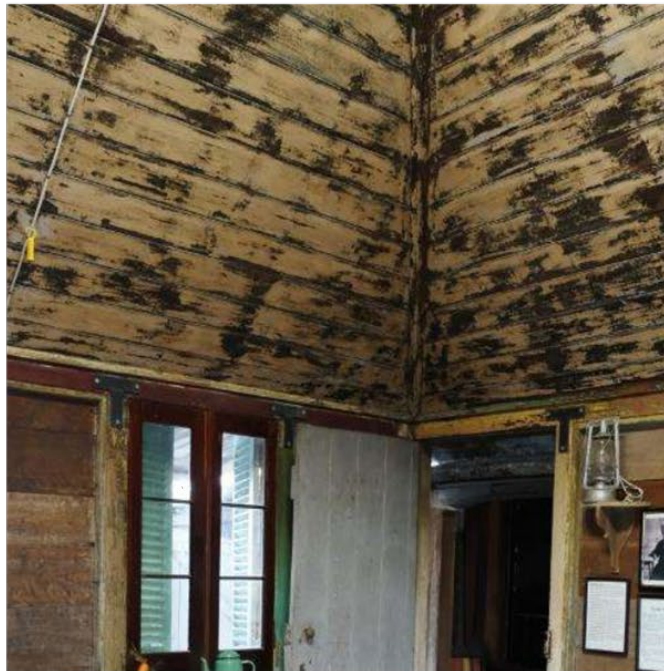
Figure 25. The ceiling of the detached kitchen, lined with unpainted, horizontally fixed beaded boards. Note the latter show evidence of being smoke or fire affected.
