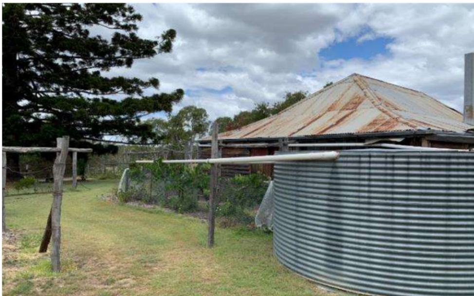
Figure 11. Exterior view of the homestead's north-west elevation. Note the hipped roof profile, the trellises adjacent to the building, and the current placement of the rainwater goods.
