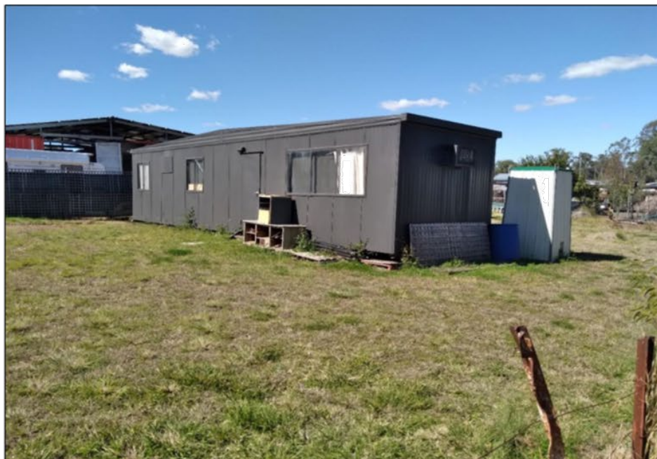
Unauthorised Dwelling with non-compliant effluent disposal
