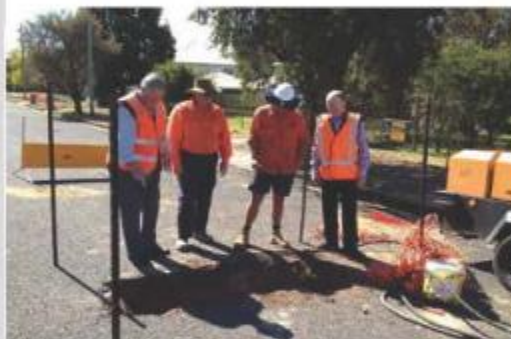
Cr Barry Green, Shane Putter, Jack Bonas, Russell Hood inspecting water sewerage infrastructure
