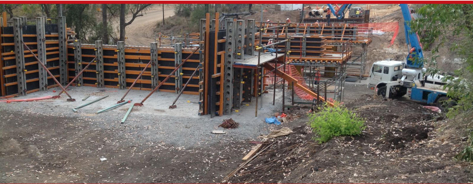
Pouring Headstocks - Stuart River Bridge, Kumbia Road
