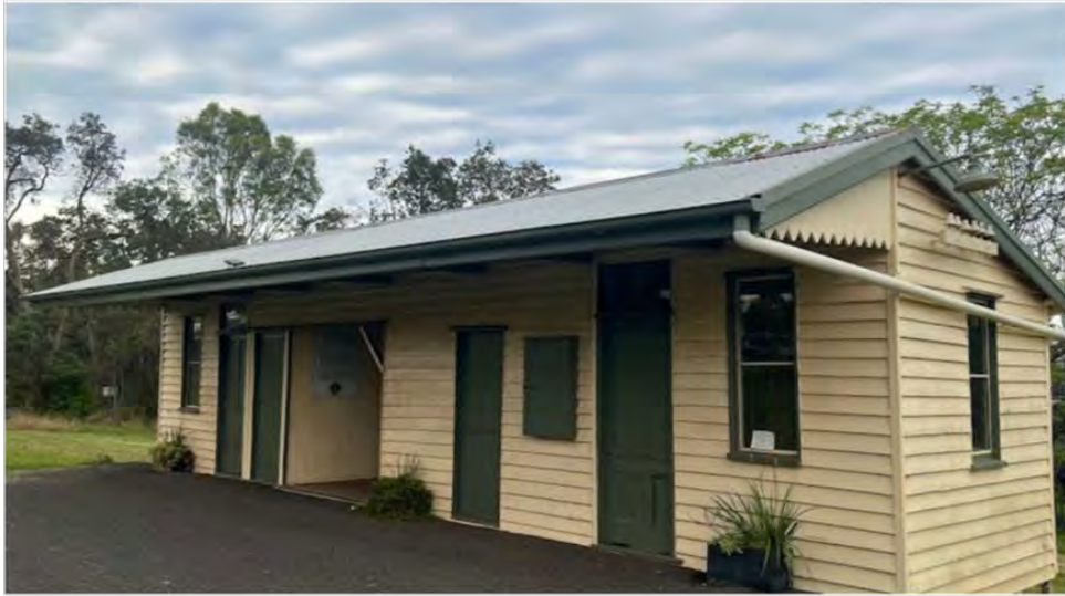
Figure 1 - Railway Station Building Wooroolin
