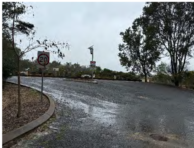
Photos of the Memerambi Waste Transfer Facility (August 2024)
