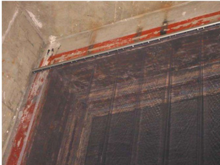
Picture 3: Mounting of 500 Series Acoustic Track.
